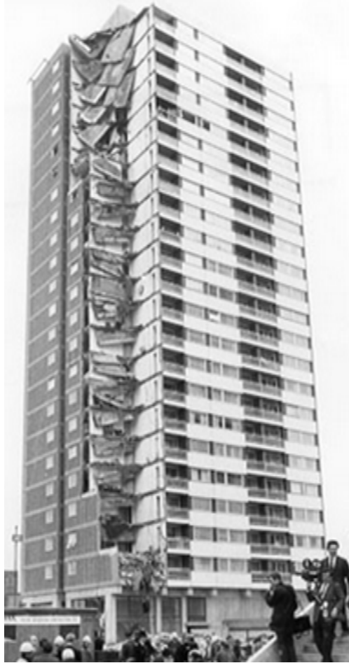
Figure 1.1: Ronan Point partial collapse (London, 1968) due to local gas explosion on the 18 th floor
