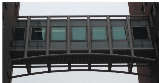
Figure 5.2: Mudd-Schapiro Link Bridge
