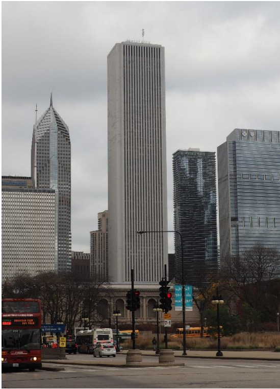
Figure 1.2 Aon Center- Chicago, IL
