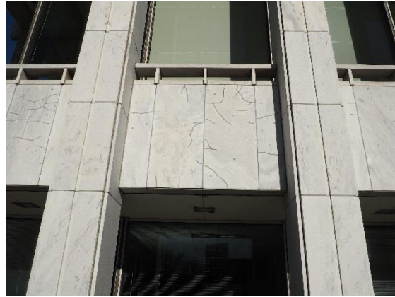
Figure 4.15 Former Life of Georgia Tower – Panel Deterioration and Repairs
