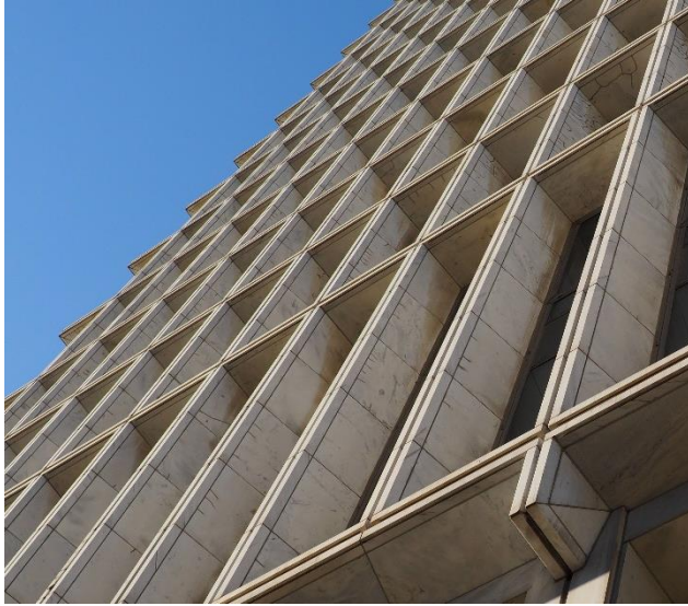
Figure 4.13 Former Life of Georgia Tower – Panel Deterioration and Repairs
