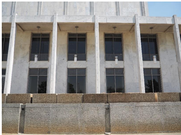
Figure 5.5 Exterior Detail – Bolted Panels
