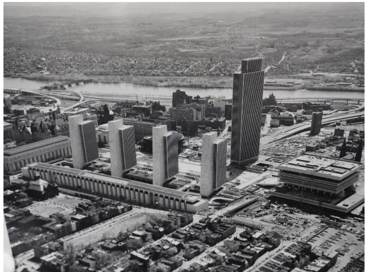
Figure 4.1 Empire State Plaza during Construction (Source NYS Library)
