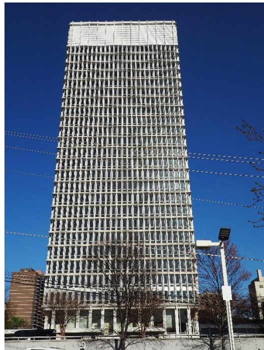
Figure 4.12 Former Life of Georgia Tower – Atlanta, GA
