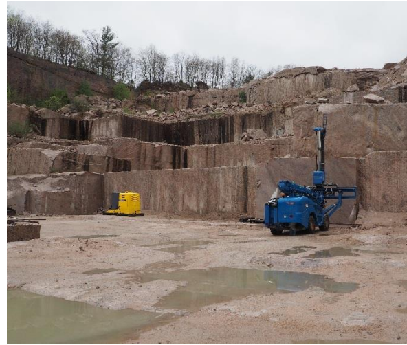
Figure 2.2 Diamond Wire – Stony Creek Quarry Branford, CT (2016)
