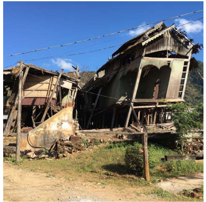
Figure 24 Tilting West Part of Haw
