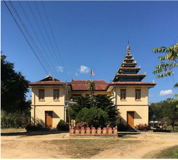
Figure 19 Lai Hka Haw (East Facade)
