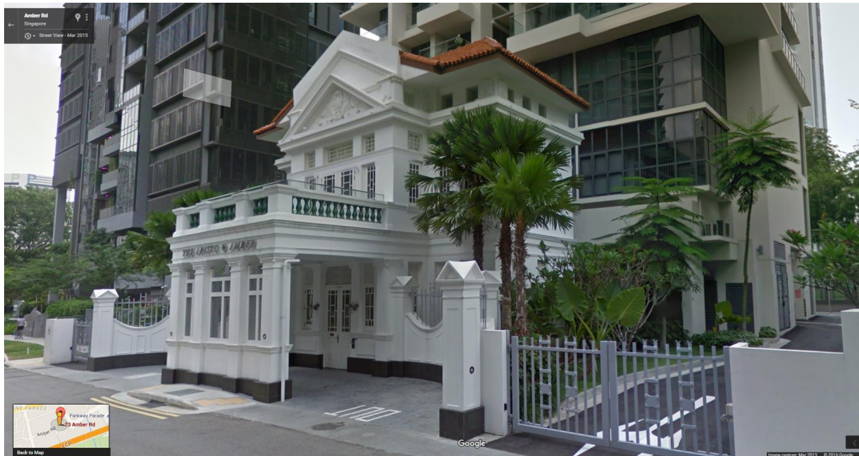
Image 6C. The retained front porch of the Butterfly House with the new condominium development.
