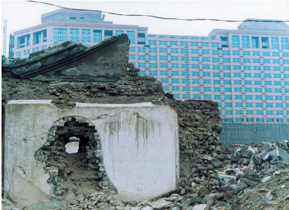
Fig. 8. ZHANG Dali (張大力) Demolition (Ciqikou, Beijing) , 1999, chromogenic color print, 100 x 150cm. From: MOMA.
