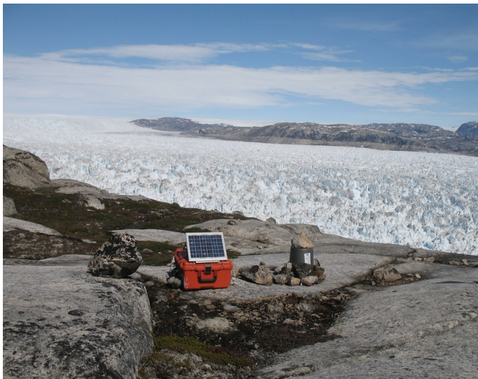
Figure 4.2: Station HM03; camera view is towards NNW. This installation is representative of the enclosure and setting of the six seismic stations used in this study. The ice visible in the station background is representative of the surface of Helheim Glacier near the calving front, and shows the highly fractured character of the lower reaches of the glacier.
