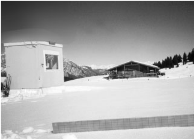
Fig. 2. The microwave station.
