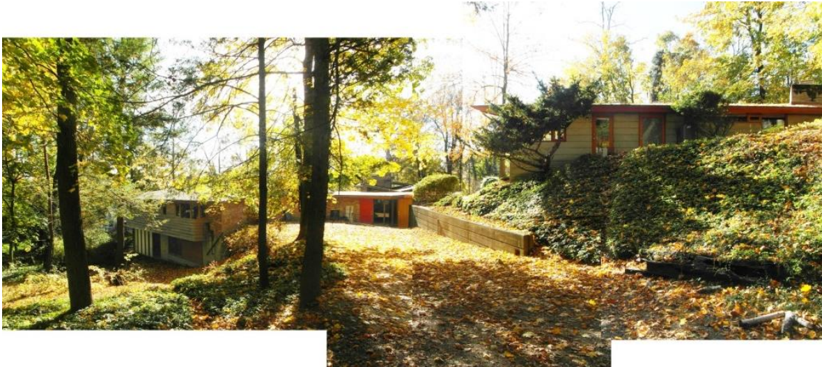
Fig. 34 – 4 Wright Way, view from the access of the site (Photo by the author)
