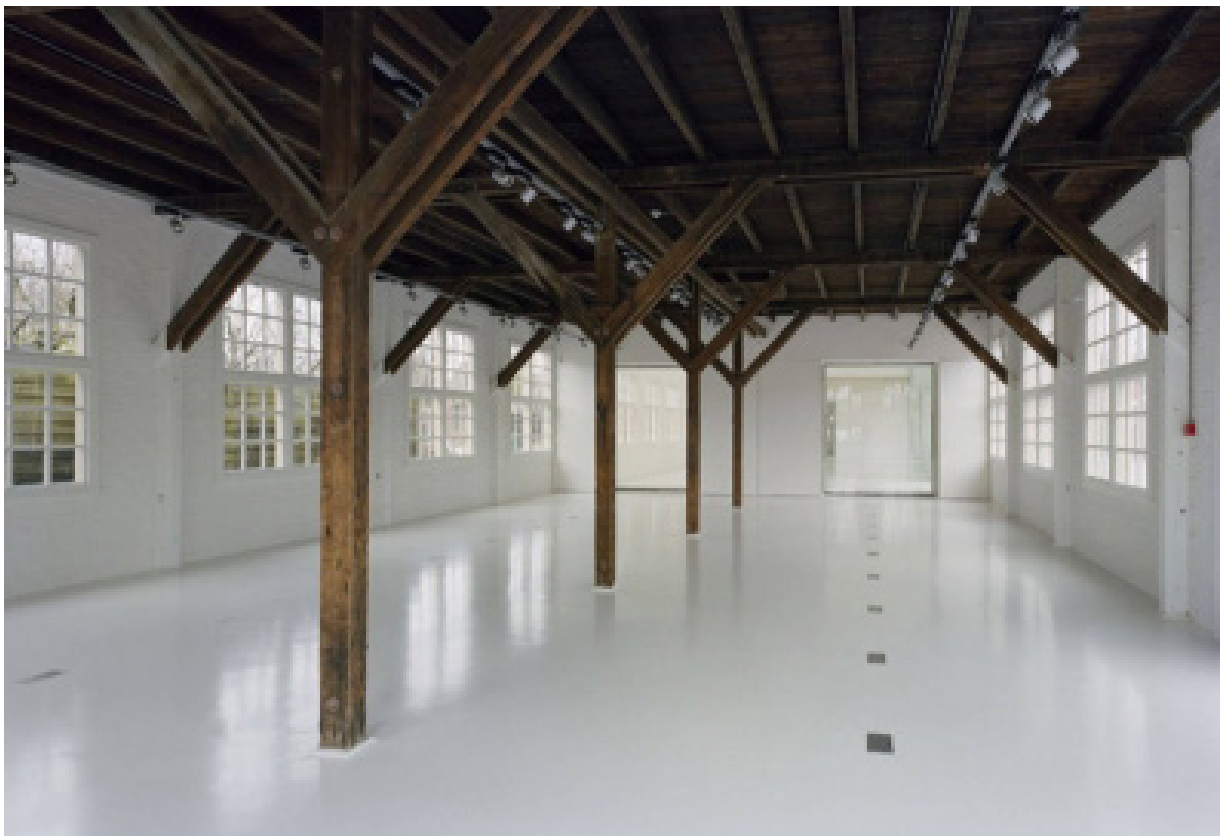
▲ 1.1: Exposed wood trusses surrounded by whitewashed masonry walls. Museum and Exhibition Hall in Veenhuizen, the Netherlands by Atelier Kempe Thill ( Casabella September 2008)
