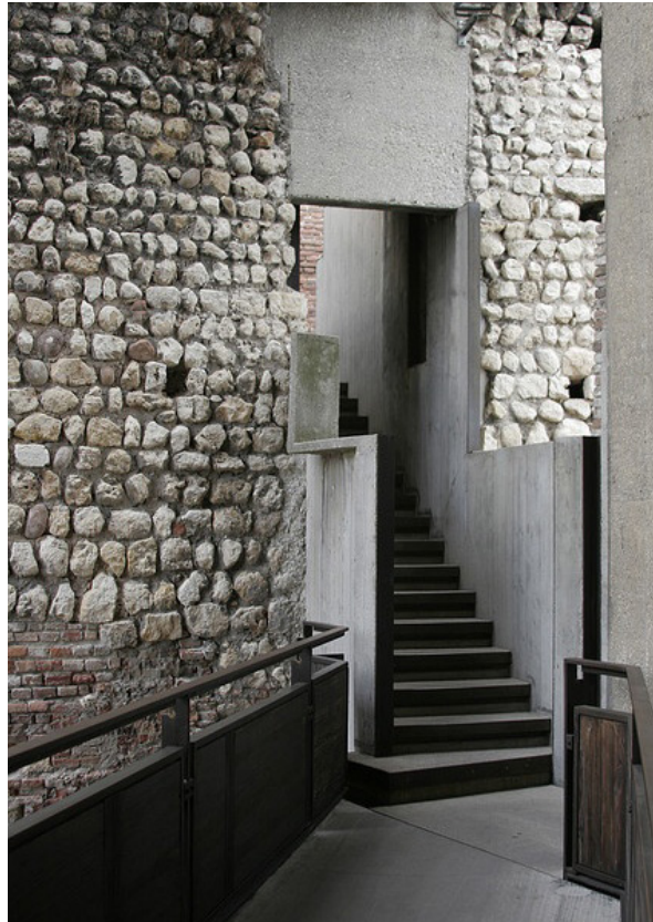
◀ 1.8: New concrete staircase inserted into existing masonry structure at the Castelvecchio Museum by Carlo Scarpa. Image via Flickr, courtesy of edwardfilms
