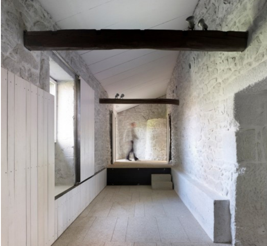
◀ 4.11: A coat of white paint applied to the thick stone walls of the Rubido Romero Foundation in A Coruña, Spain by Abalo Alonso Arquitectos ( AR , December 2013)
