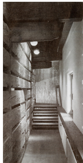
◀ 4.5: Exposed wooden beams with contemporary steel supports. Diocesan Museum in Eichstatt, Germany by Karljosef Schattner. 1977-1982. ( Detail , May 1985)
