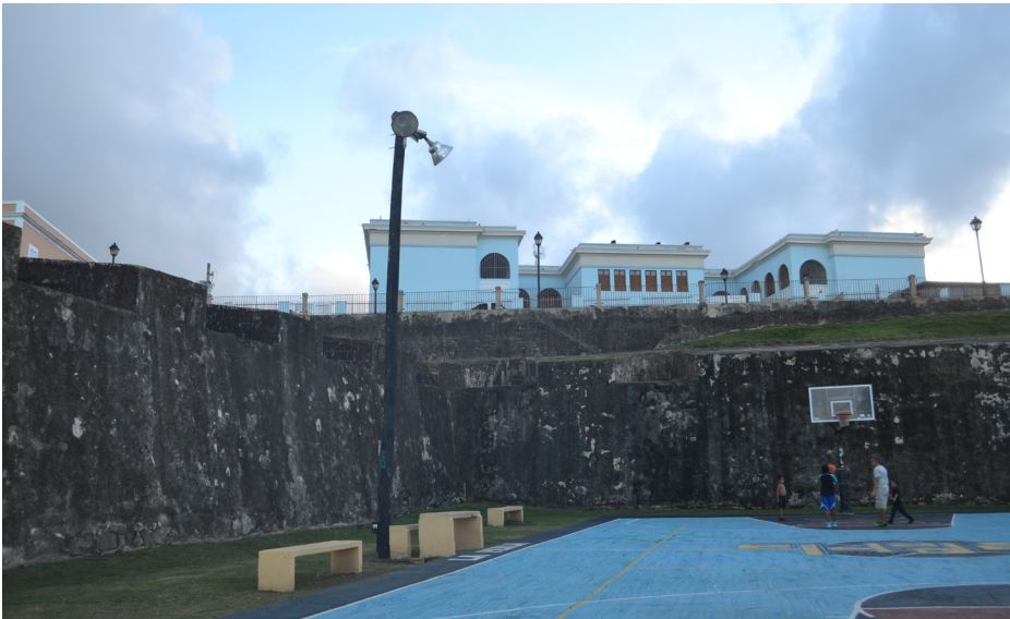
Figure 37. Lincoln Elementary School, La Perla basketball court in the foreground.
