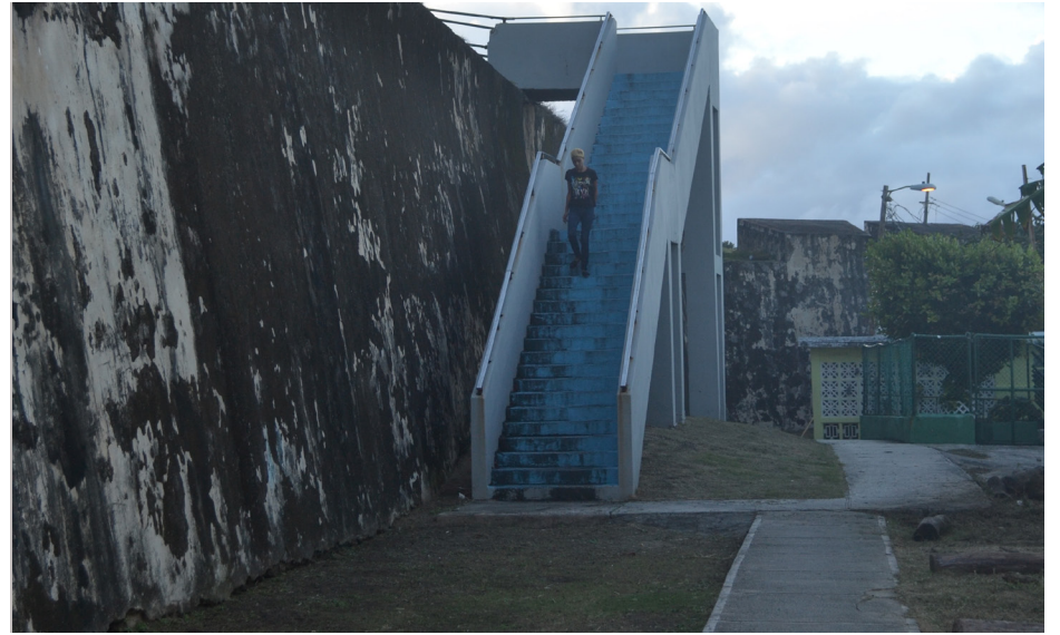
Figure 19. The other pedestrian stairs leading into La Perla.
