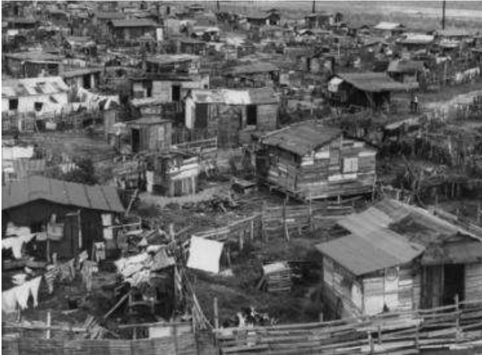
Fig. 133 Corea slum, Cantera peninsula in San Juan, under demolition
