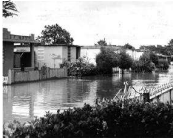
Fig. 132 Flooded section H of Puerto Nuevo
