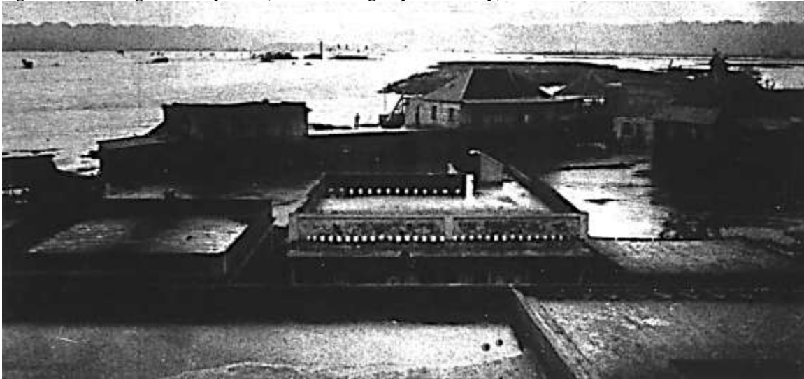
Fig. 6 Life saving port station destroyed, Arecibo
