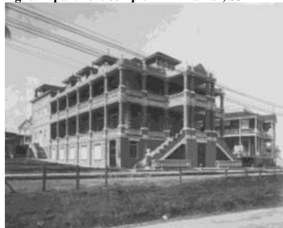
Fig. 69 Apartment complex in Miramar, SJ
