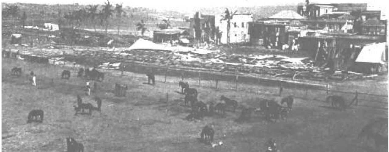
Fig. 27 Damage to the American mounted troop's stables, undisclosed location
