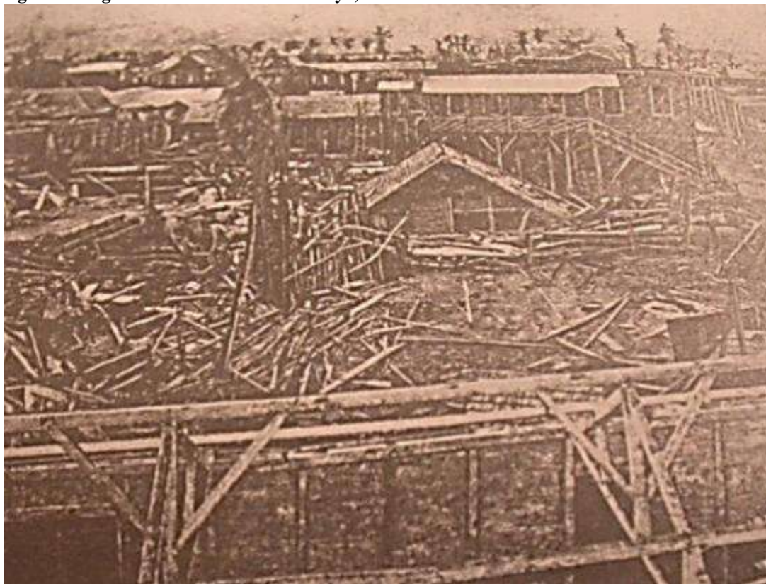
Ruined wood structures photographed from Mr. McCormick's rooftop. Image: (Rosario Rivera, 2000a, p.40).
