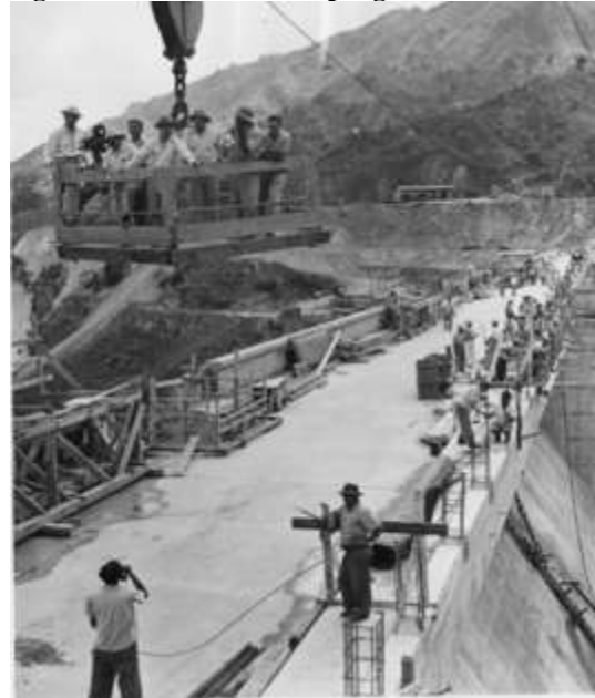
Fig. 113 Caonilla Dam in progress
