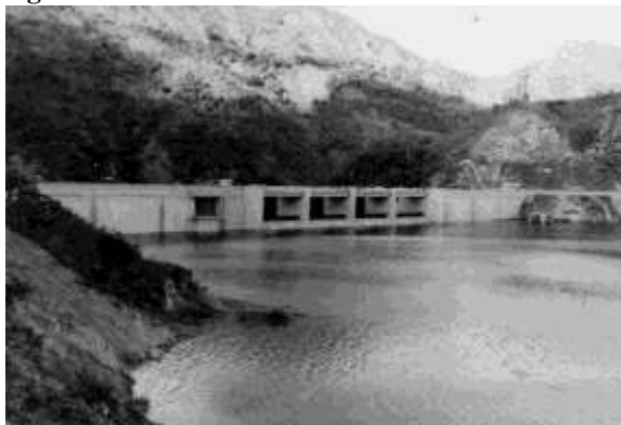
Fig. 114 Finished Caonilla Dam
