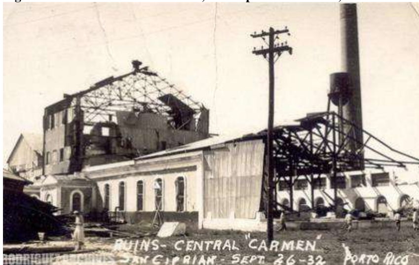
Fig. 88 "Ruins at Central 'Carmen', San Ciprián Hurricane, Porto Rico"
