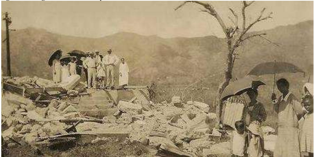
The hurricane razed a concrete and brick house to its foundations, image by (Anonymous, 1928c).
