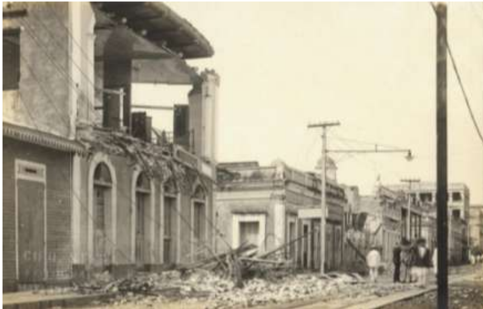
Fig. 46 Earthquake destruction in Mayagüez
