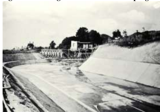
Fig. 115 Toro Negro 2 overflow canal in progress
