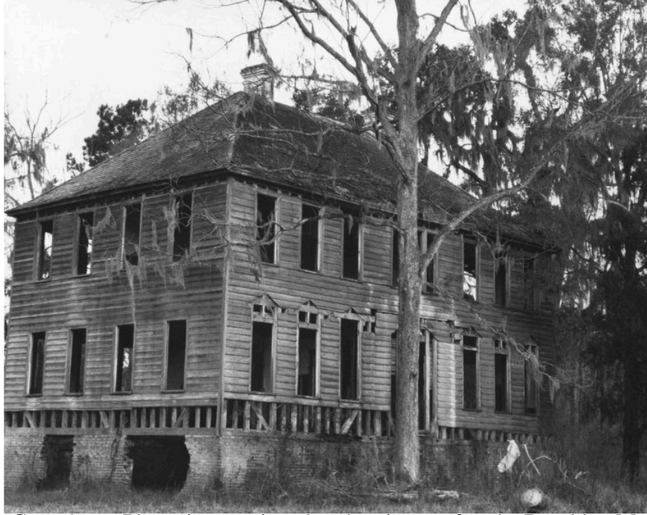
Figure 1.3: Cane Acres Plantation continued to deteriorate after the Brooklyn Museum removed woodwork from its dining room. Taken in 1946, this photograph shows the house just before it collapsed.
