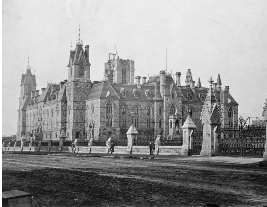
The West Block of Parliament under construction, view looking West. 98
