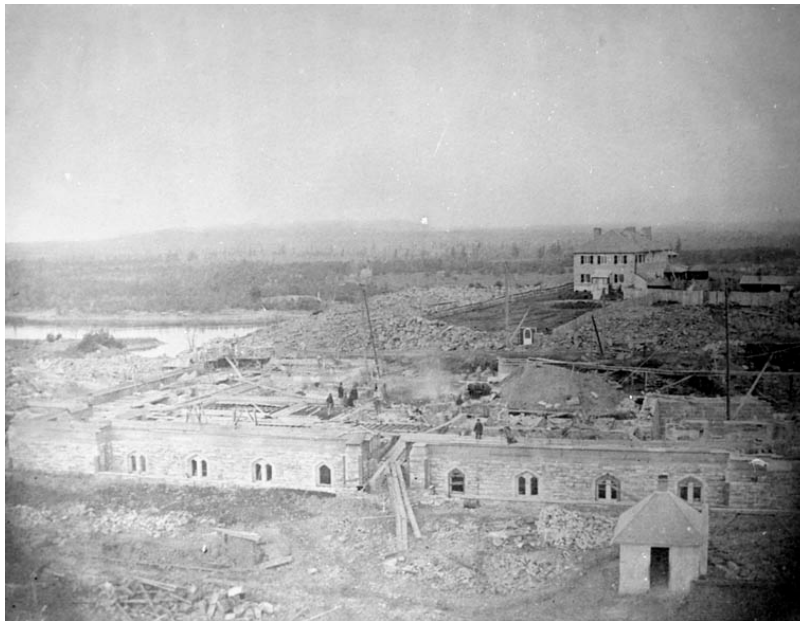
West Block of Parliament Buildings in the early stages of construction, 1861. 97
