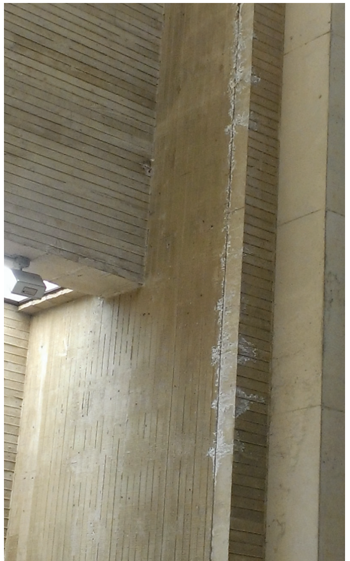
Orange County Government Center - Water Infiltration and Structural Repairs
