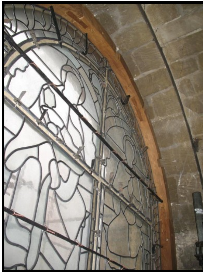
Figure 67. Protective glazing done with the major lead lines of the window for better aesthetics. Image from http://vidimus.org/issues/issue-27/news/
