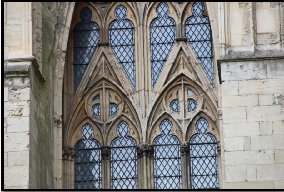
Figure 66. Quarry pattern protective glazing on York Minster Cathedral. Image from personal collection.
