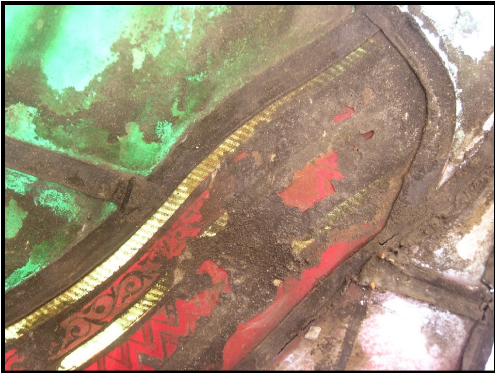
Figure 49. Weathering crusts on the surface of the glass. Image courtesy of Drew Anderson.
