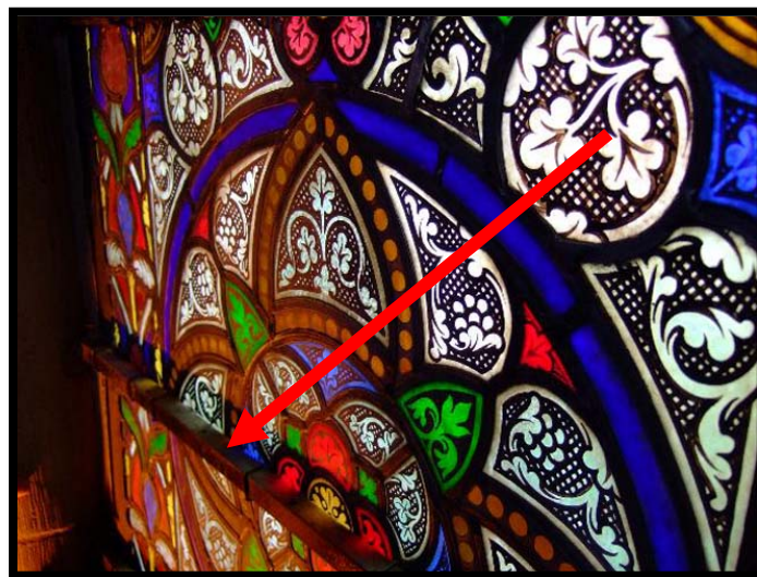
Figure 8. A saddle bar and ties used for supporting a stained glass window. Image from CVMA Glossary. 2010.
