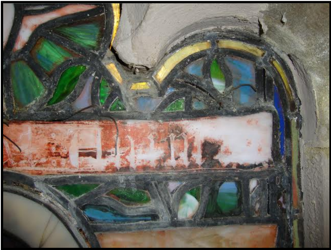
Figure 36. Paint deterioration on “The Annunciation” window by Otto Heinigke, ca. 1890, shown in reflected light. Image courtesy of Julie Sloan.
