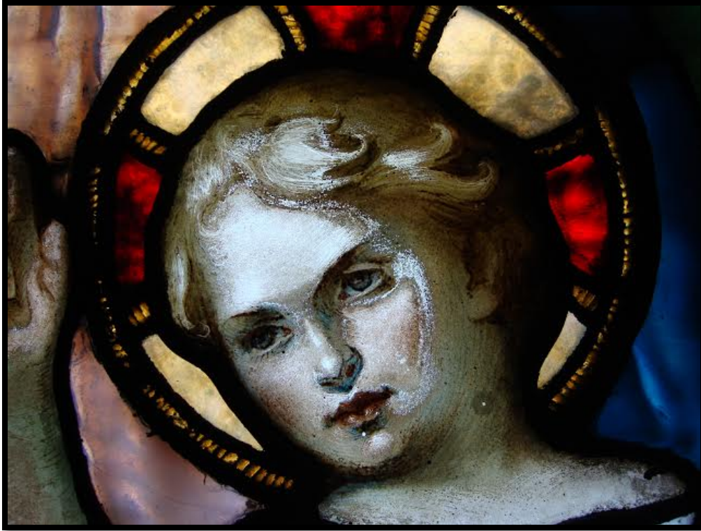
Figure 37. Paint loss on “Adoration of the Magi” by Harry Eldredge Goodhue, ca. 1898, shown in transmitted light. Image courtesy of Julie Sloan.
