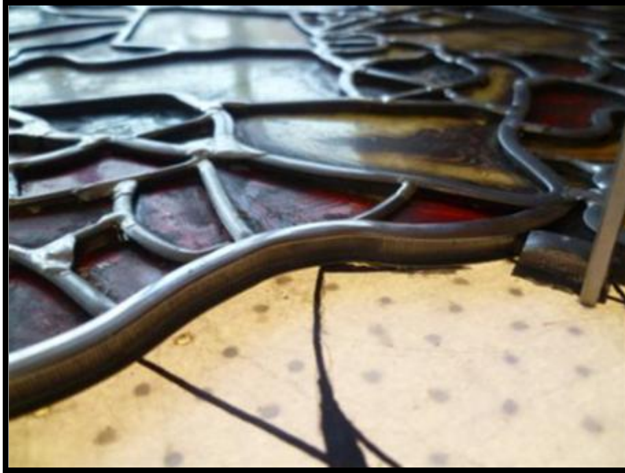
Figure 6. Lead came in a stained glass window. Image from The York Glaziers Trust, "Illustrated Glossary."
