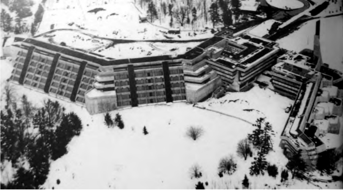
Fig. 0.4 John Andrews, Scarborough College, Toronto, 1965: an early and celebrated instance of megastructures
