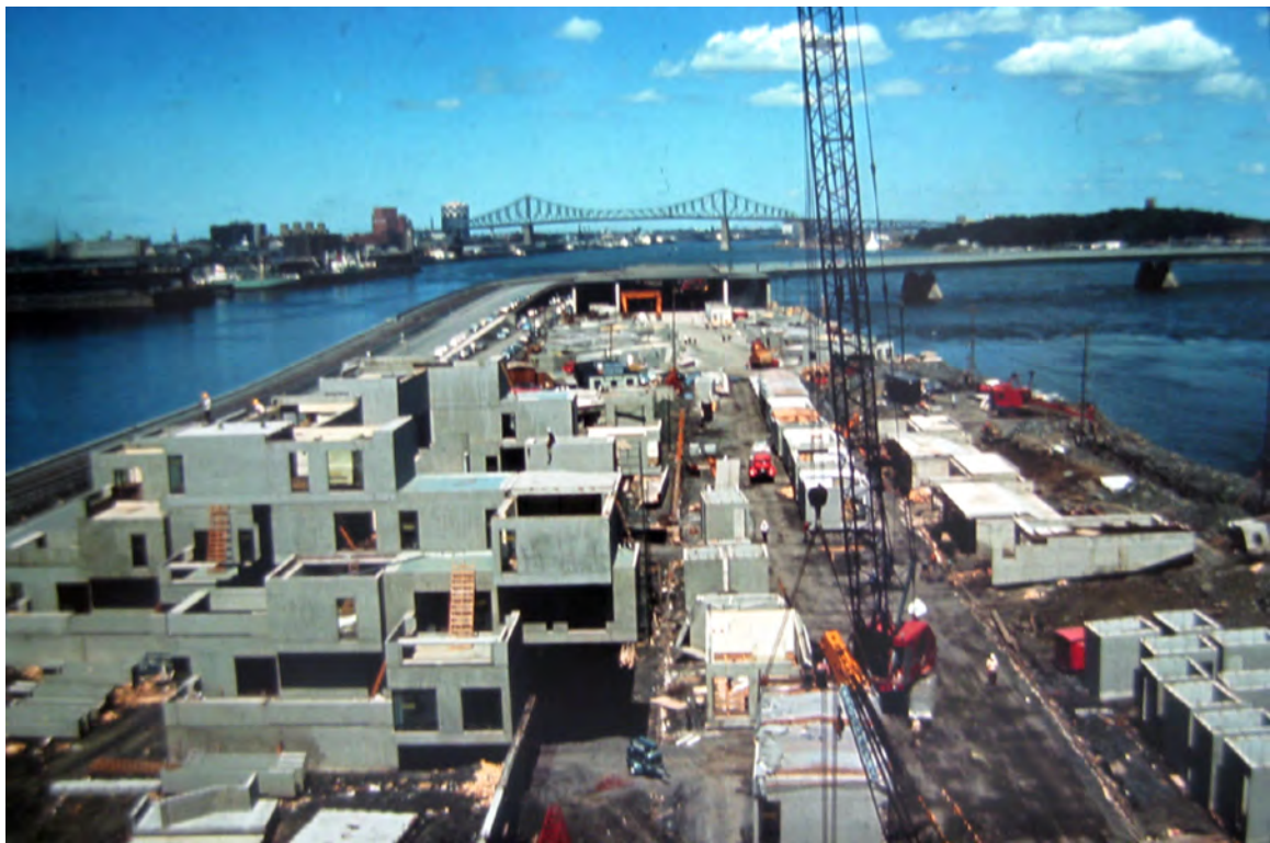
Fig. 6.13 “Assembly-line” construction, circa 1966
