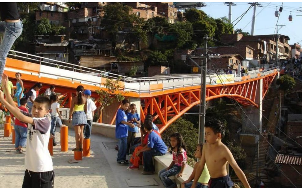
Figure 9. Bridge between Andalusia and La Francia barrios. Source: EDU
