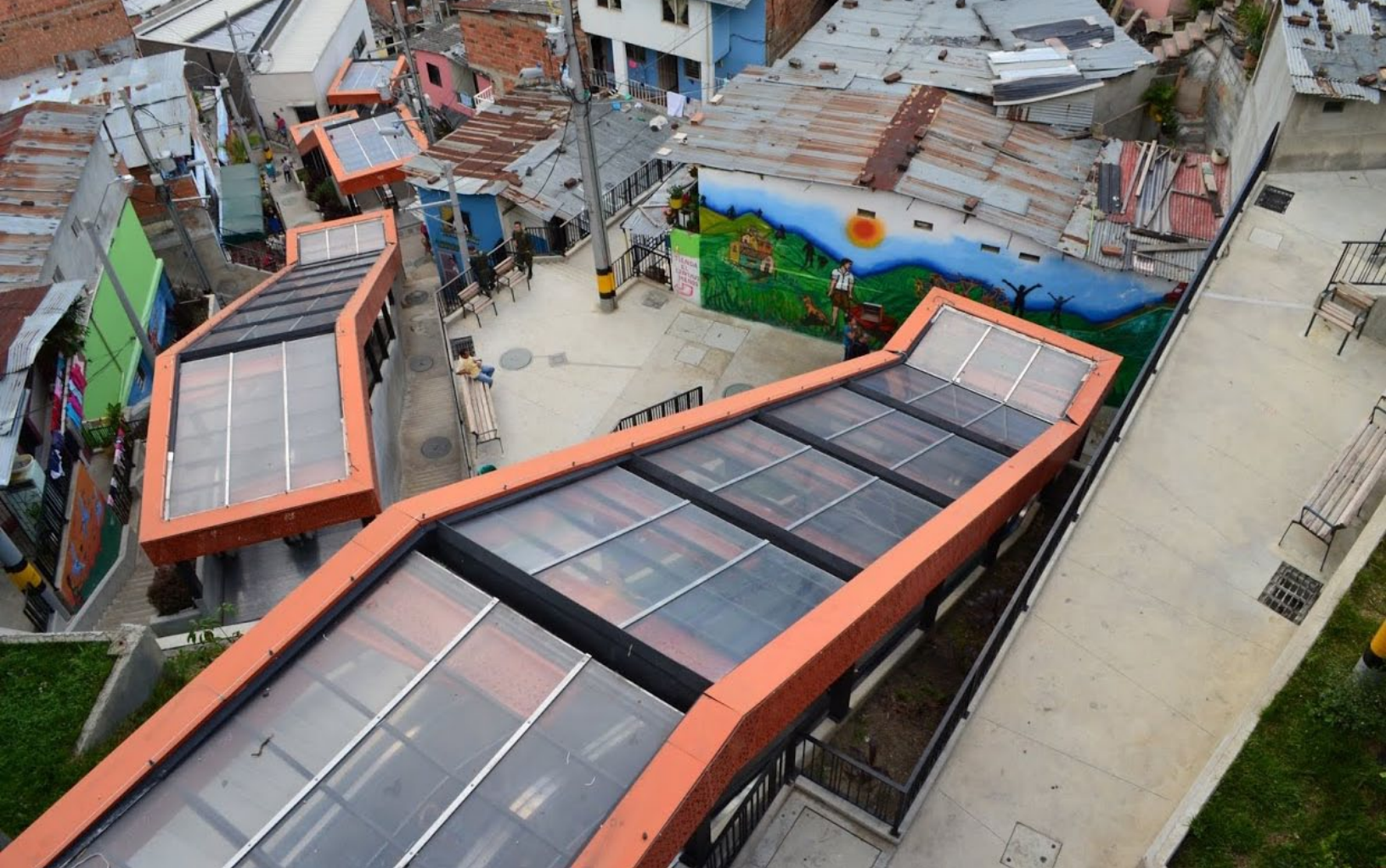
Figure 14, Comuna 13 Escalator project. Source: Jet Richardson
