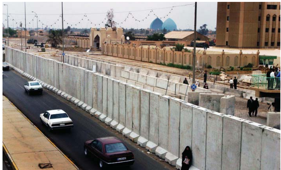
The walls of the Green Zone. Image source: media.worldbulletin.net
