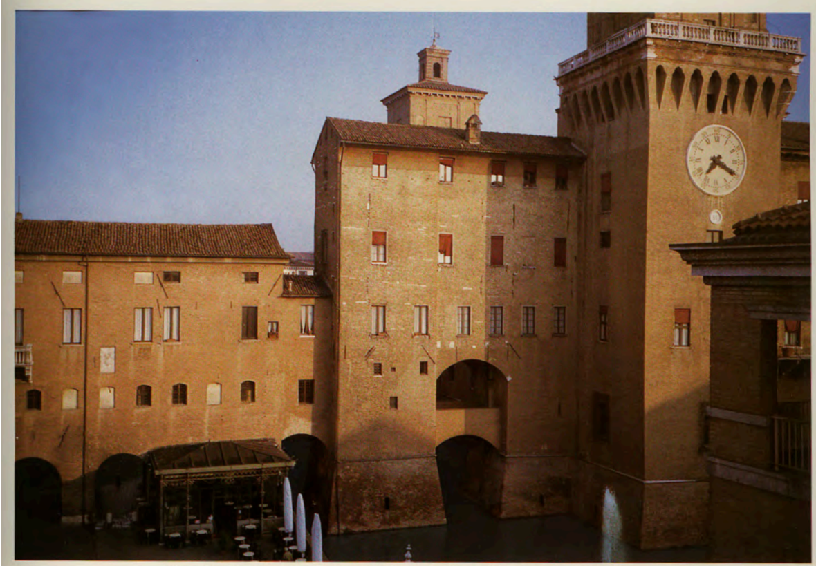
Fig. 6.7 View of the Via Coperta and Ravelin and Tower of the Castello Estense, Ferrara. (Ballarin, 2002)
