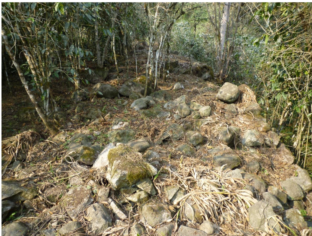
Figure 4.16. The upper portion of one the large wall segments at Capillayoq. Note the drop-off down to the gully on the right of the picture.
