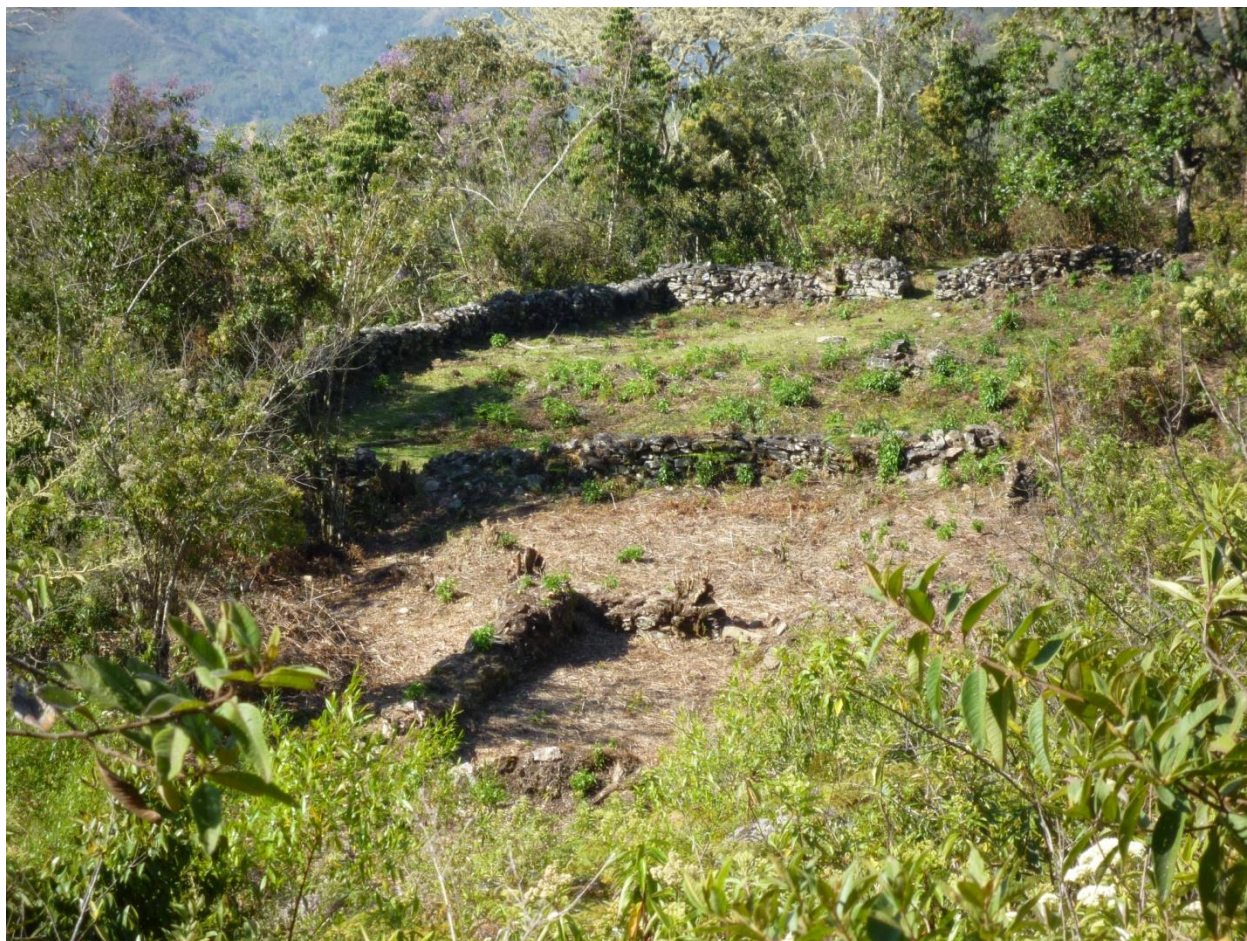
Figure 7.8. Image showing enclosure S-059, seen looking east. The smaller structure visible in the foreground is S-107.
