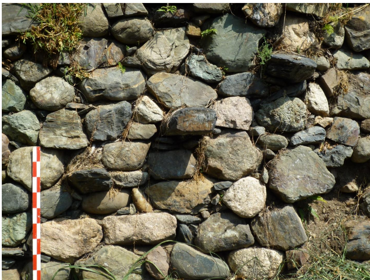
Figure 4.5. Detail of well-preserved set of tenon-steps running diagonally along a terrace wall at Cangrehuyoc.
