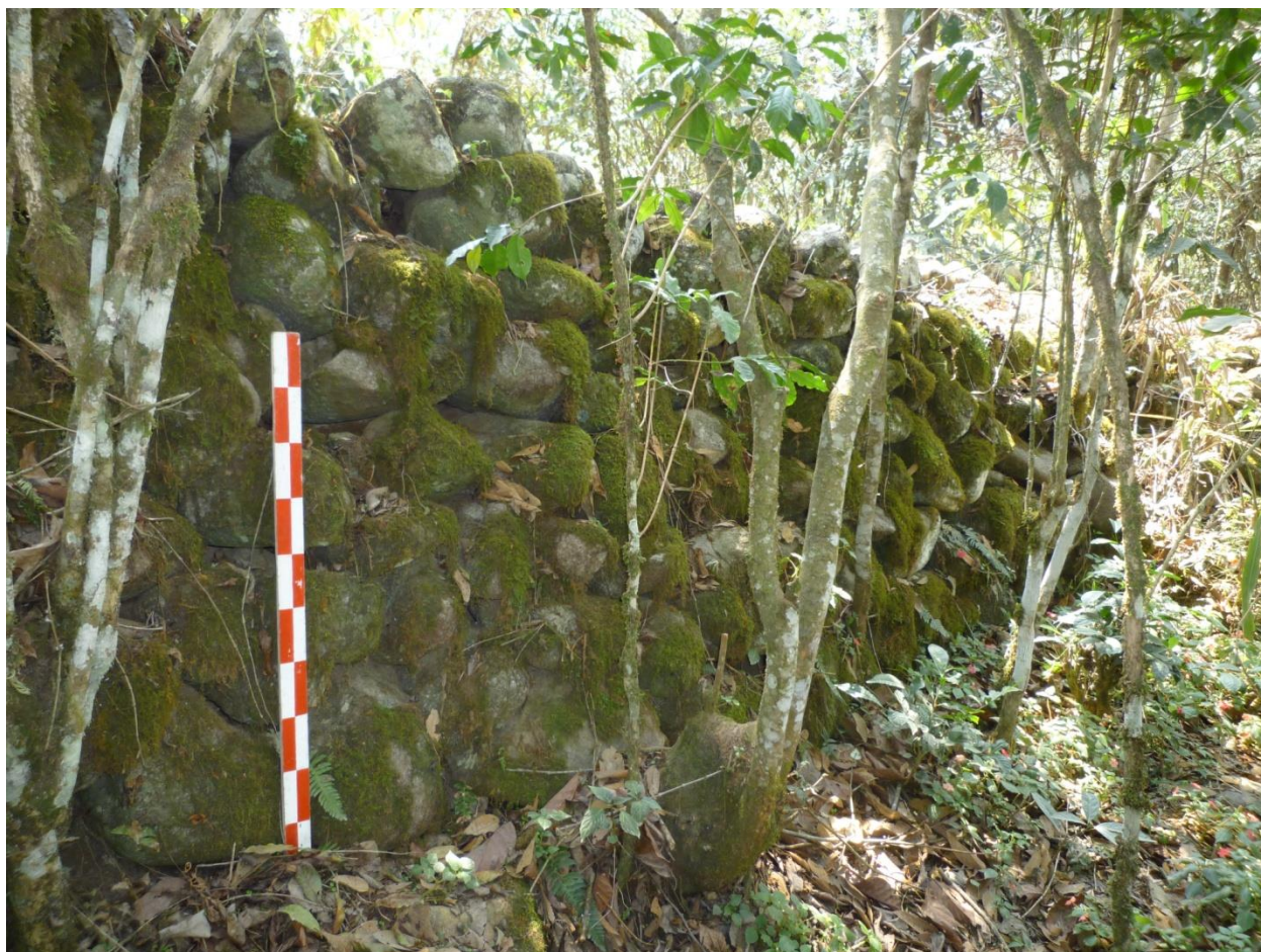
Figure 4.15. A portion of the large retaining wall at Capillayoq.
