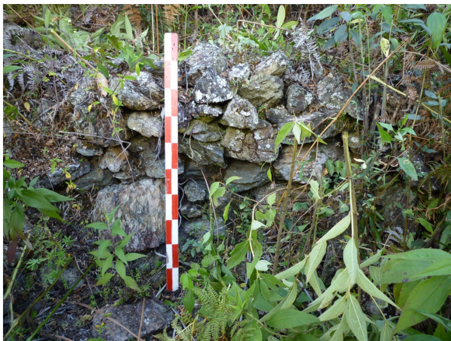
Figure 5.10. Portion of retained wall along road at Qochapata, seen looking southwest.
