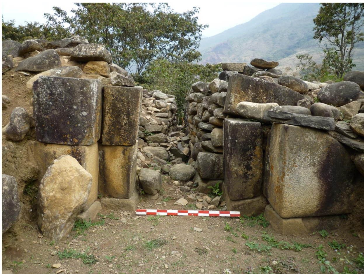
Figure 4.3. A surviving portion of a double-jamb doorway, located on the southern flank of the courtyard. Note the finely carved ashlar masonry.
