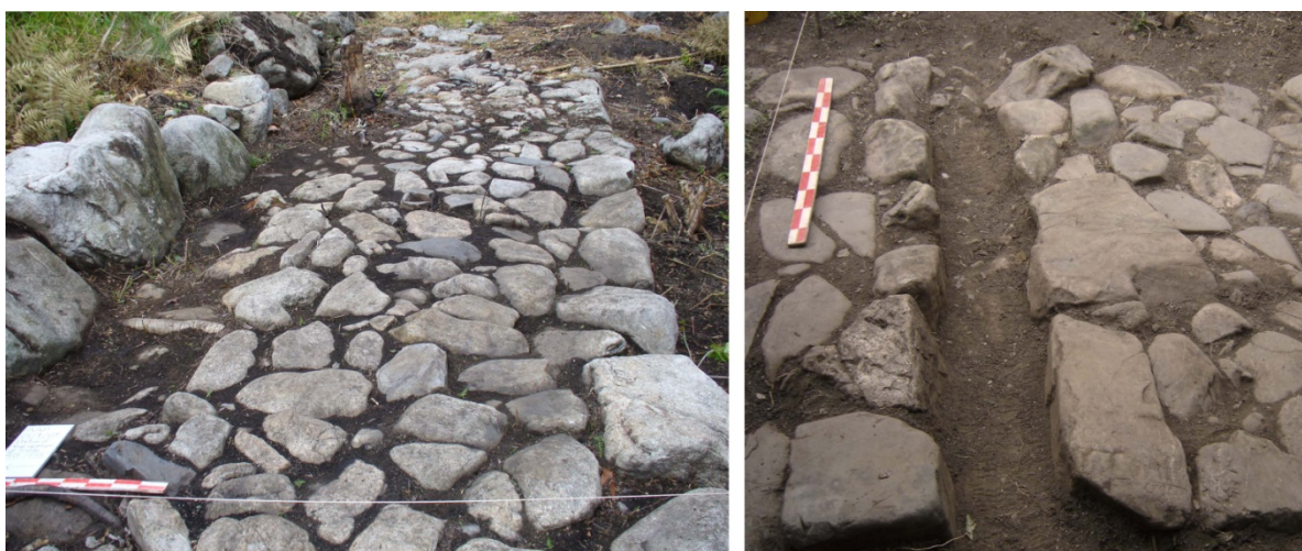
Figure 5.5. Photographs of paved surface of Road Segment A (left) and of well-preserved drainage channel in Road Segment E1 (right).
