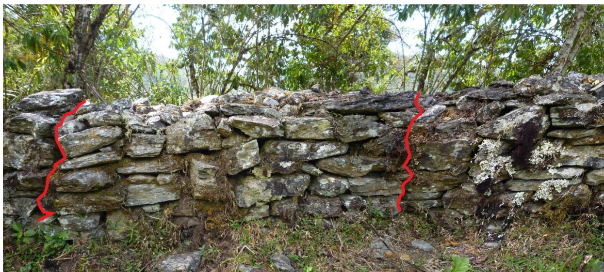
Figure 7.10. Panoramic montage of the interior face of the northern wall in S-059, with the abutting parts of the construction segments highlighted. The wall in the image is approximately one-meter in height.
