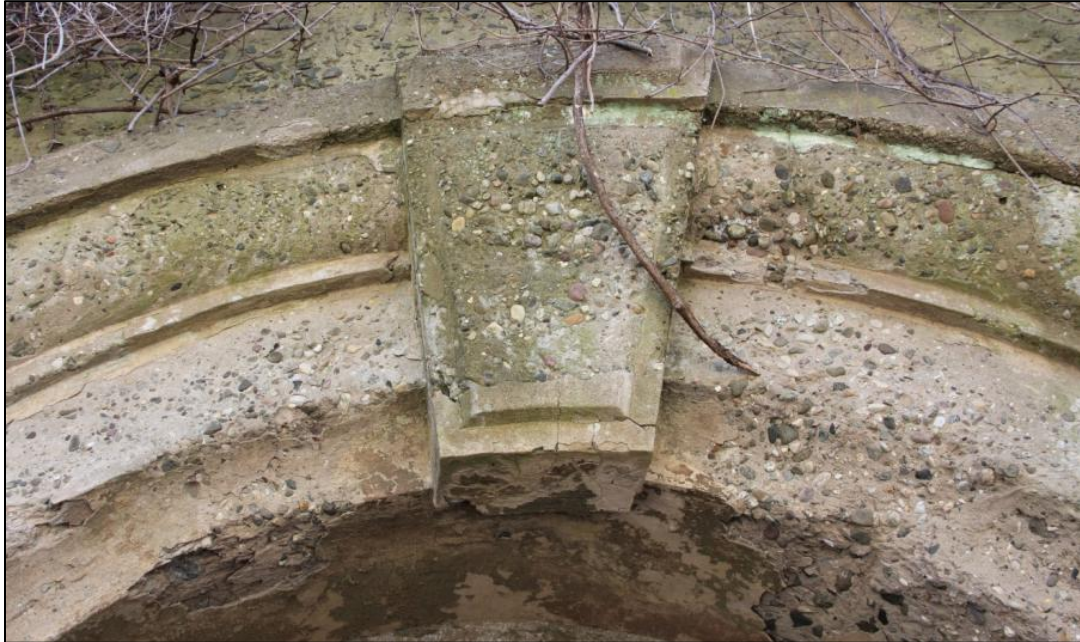
Figure 53: North entrance of tunnel, showing decorative concrete moldings and keystone (2012)
