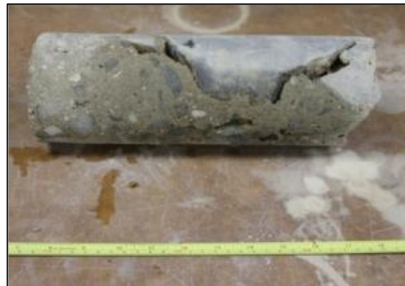
Figure 86: Torpedo Magazine 8 Core (1875/6), note the large aggregate and surrounding voids
