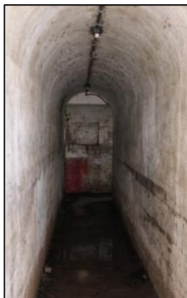
Figure 20: Entrance Tunnel Main Magazine (2012)
