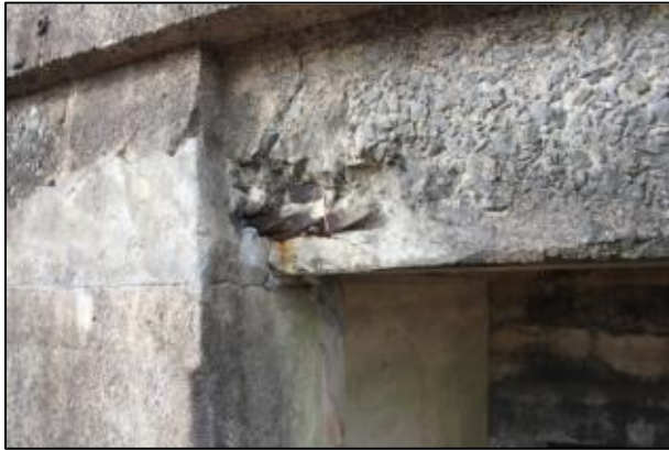
Figure 78: Battery Mahan 1 Upper, southern extension, showing reinforced concrete
