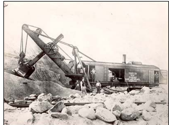
Figure 120: Steam shovel, Phoenix Sand and Gravel Company, Port Washington, N.Y., 1910 (courtesy of Port Washington Public Library)
