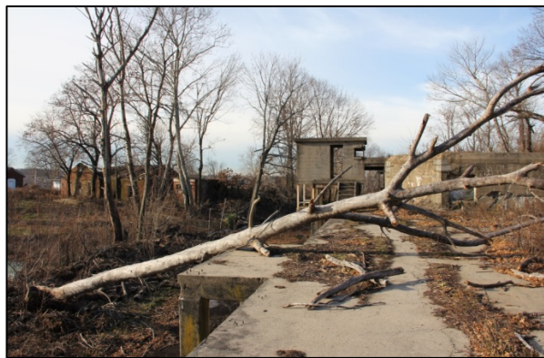
Figure 70: Battery Mahan 1 showing tree knocked over by Hurricane Sandy (2012)
