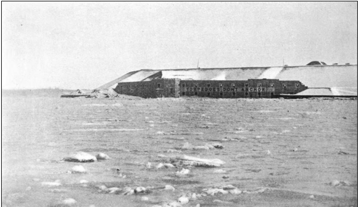
Figure 35: Water Battery and the reconstituted bluff behind shielding the Endicott Batteries (Abbott, 1904, p. 17)
