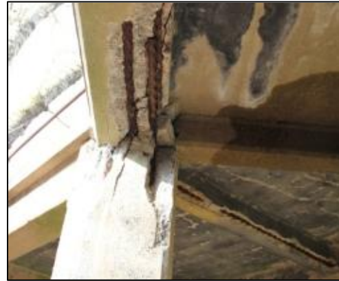
Figure 79: Battery Summer 1 Lower Core, southern extension, showing reinforced concrete
