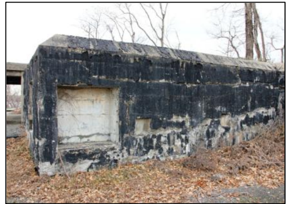
Figure 62: Bituminous coating at Battery Mahan 2 (2013)
