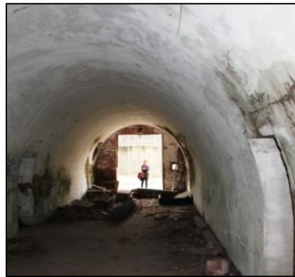
Figure 28: Torpedo Magazine, showing two doorways cut into the side walls (2013)
