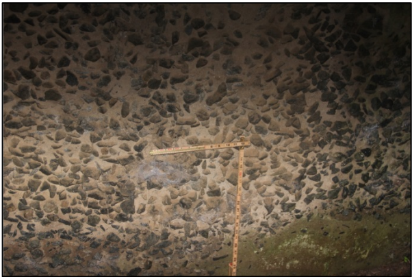
Figure 76: Coarse concrete foundations of Battery Graham 1 (1892-1897)
