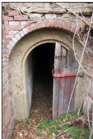
Figure 32: Magazine entrance of the surviving 1870s Battery (2013)
