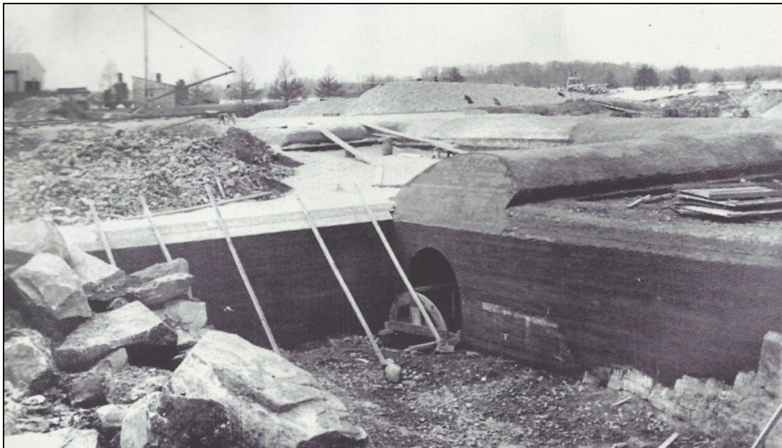
Figure 52: Construction of the batteries and magazines at Fort Totten, ca. 1890s, showing wooden formwork (Bayside Historical Society Collection)
