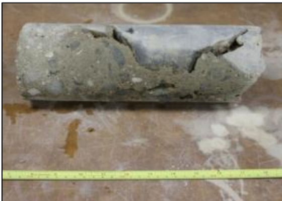
Figure 85: Torpedo Magazine 8 Core (1875/6), note the large aggregate and surrounding voids
