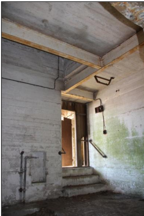
Figure 57: Extension of Battery Sumner 1 showing the rolled steel I-beam supports (2013)
