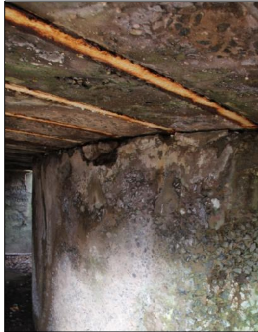
Figure 56: Battery Graham 1, ceiling showing rolled wrought iron beam and concrete infill ceiling surrounding the gun foundations. (2012)
