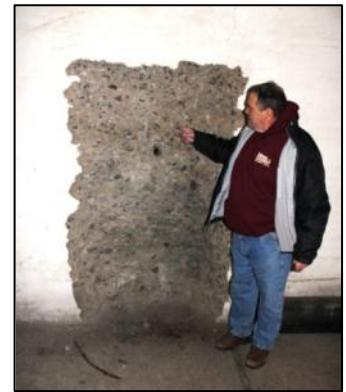
Figure 29: Torpedo Magazine, showing a partially cut doorway in the sidewall (2013)
