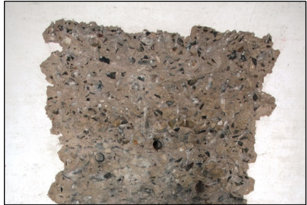
Figure 73: Partially completed doorway cut through the sidewall at Torpedo Magazine 3 (1873-1876)
