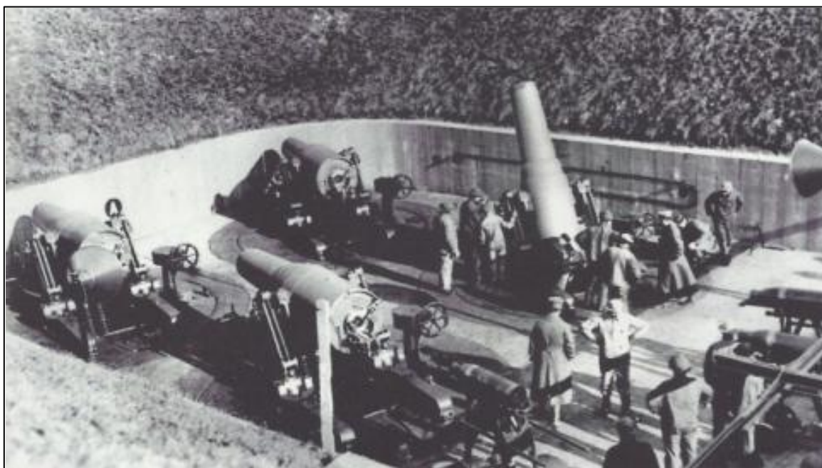
Figure 47: Battery King, showing one of the Abbot Quad mortar pits ca.1920 (Fort Totten Museum Collection)
