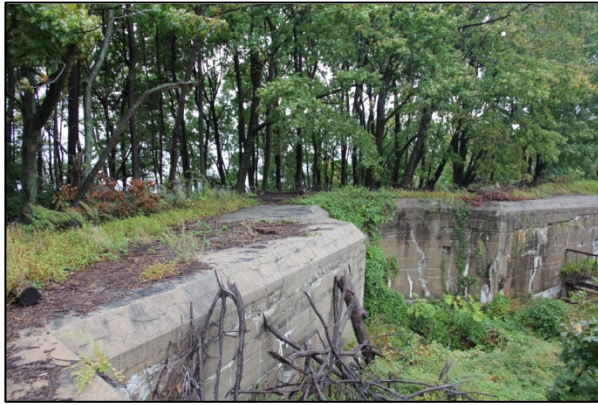
Figure 66: Battery Mahan 1, showing trees colonizing the earthen ramparts in front of the blast apron (2012)
