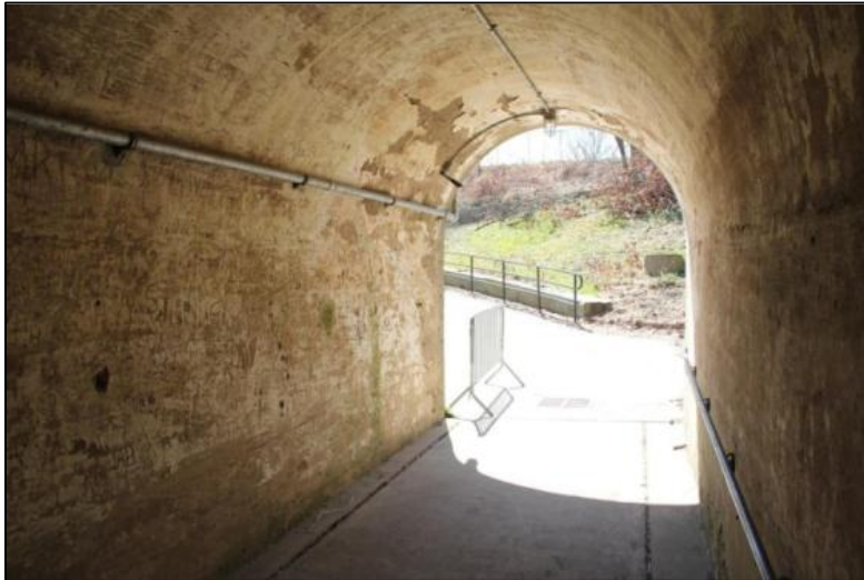
Figure 23: Tunnel interior, showing graffiti, and south entrance (2013)
