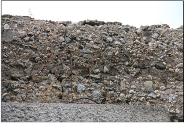
Figure 72: Coarse infill concrete used at the Water Battery (1862-67)
