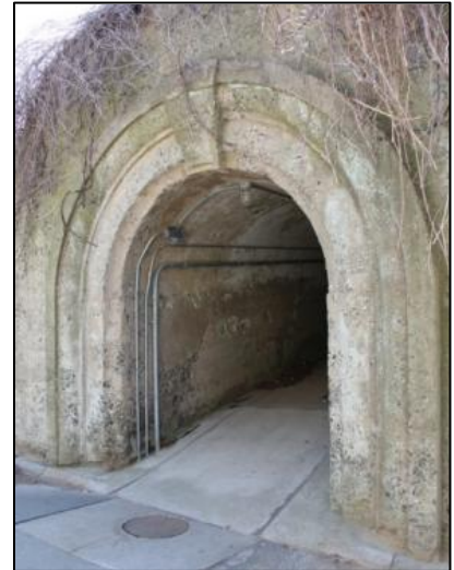
Figure 24: North entrance of tunnel, showing decorative concrete moldings (2013)
