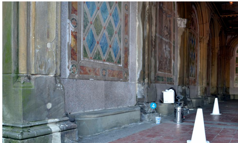
Bethesda Terrace arcade column base (east wall)
