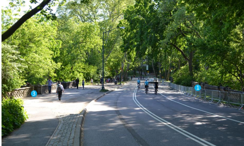
Balcony Bridge (looking south)
