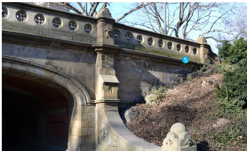
Dalehead Arch balustrade (east elevation)
