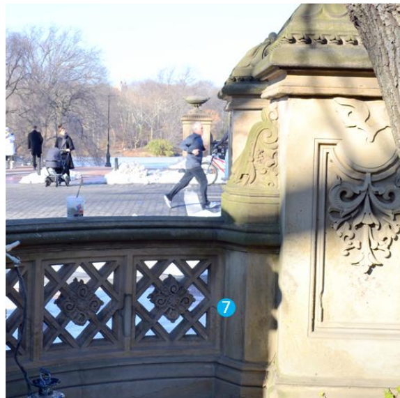
Bethesda Terrace balustrade (upper terrace on west side)
