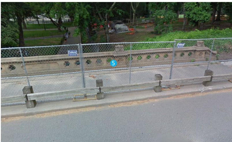
Driprock Arch west balustrade (side facing east)
