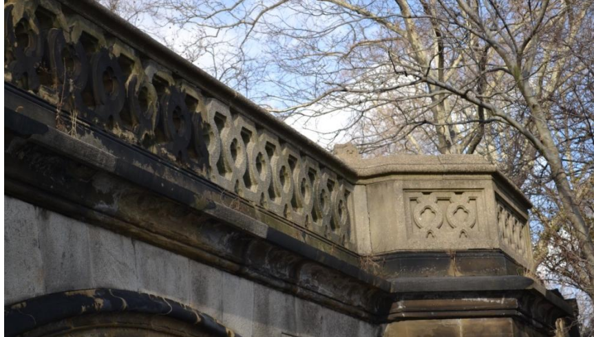
Figure 1.12: Eastern balustrade of Balcony Bridge showing use of cast-stone for replacement
