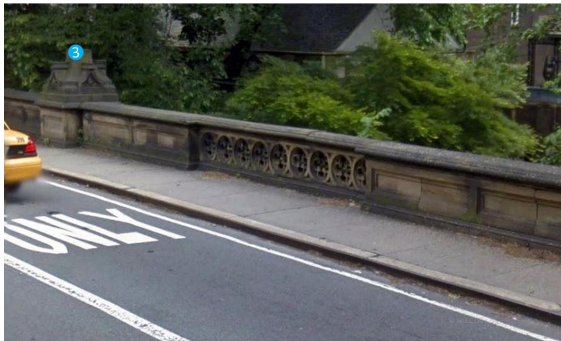
Denesmouth Arch south balustrade (side facing north)
