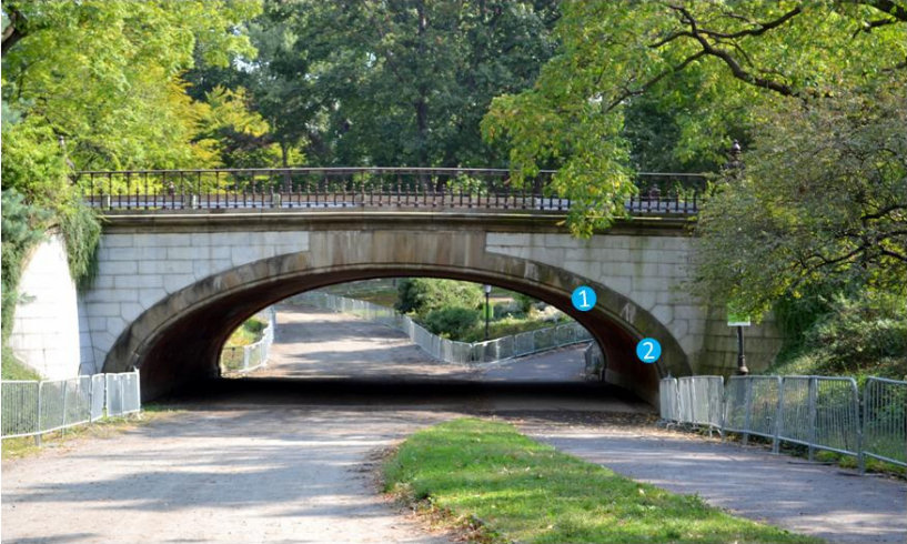
Winterdale Arch (west elevation)
