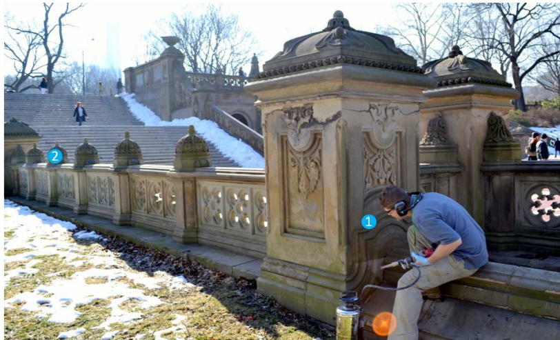
Bethesda Terrace pier and balustrade (lower terrace on east side)
