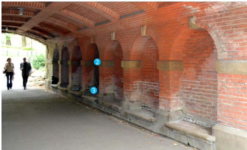
Willowdell Arch (north interior wall)
