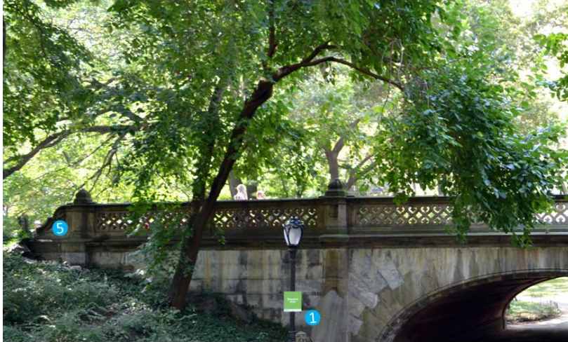
Greystone Arch (east elevation)
