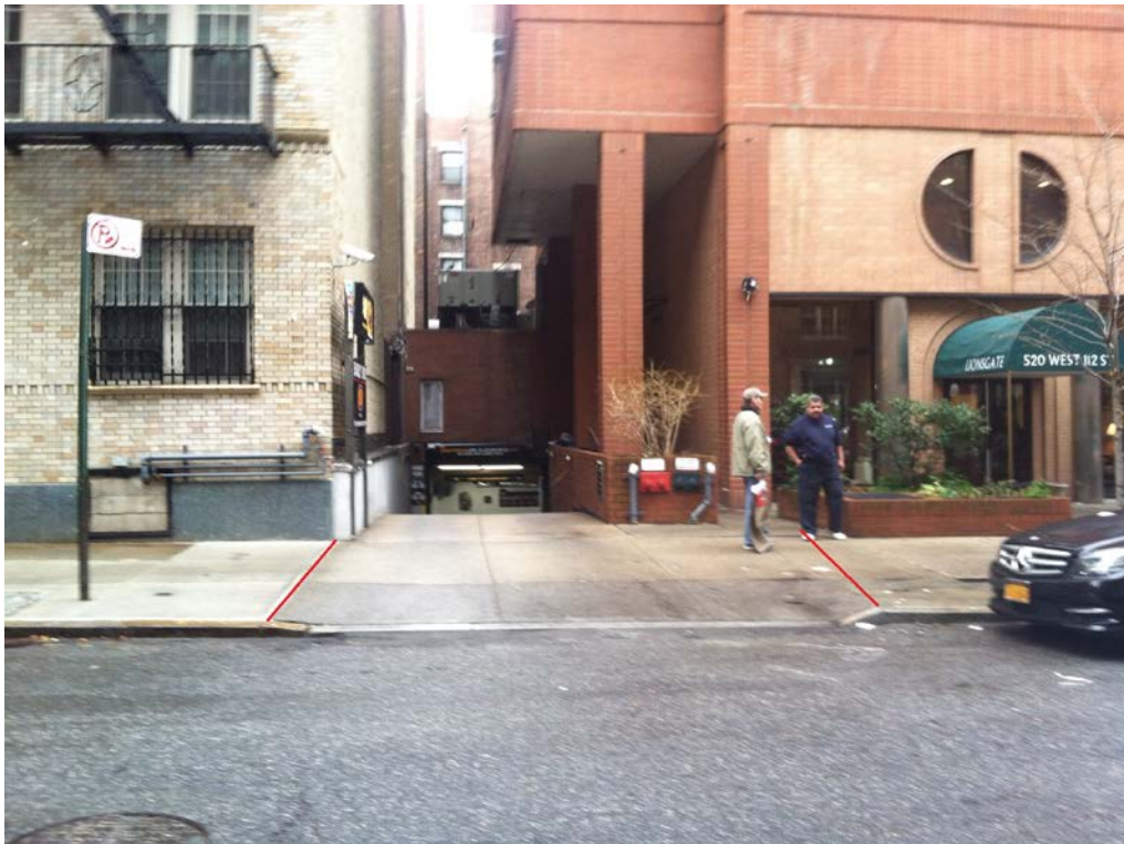
Figure 3. The red lines indicate where measurement for the curb cut began and ended for each curb cut.
