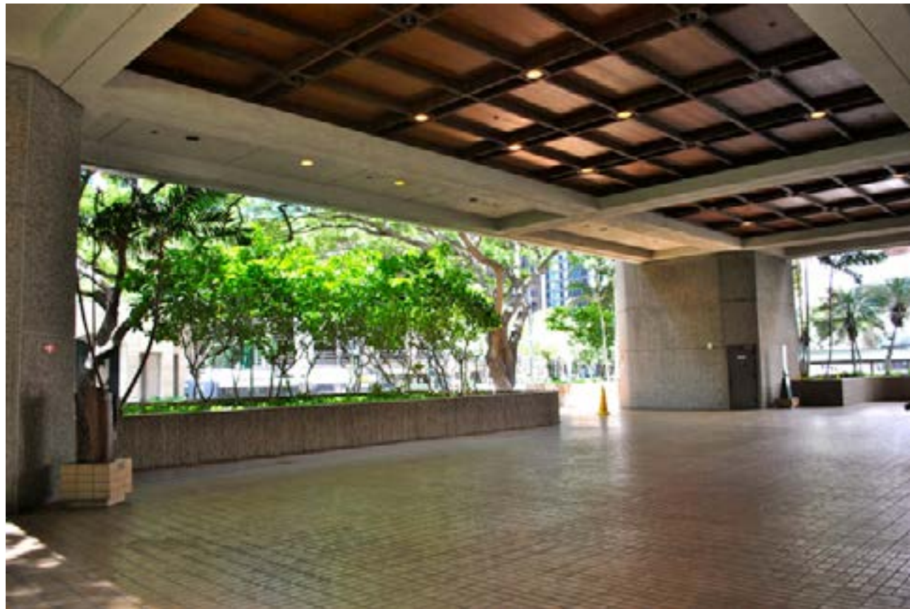
Images 37: An interior view of the Kealiko-lani Hale Building, Honolulu. Personal photo by author, September, 2012.
