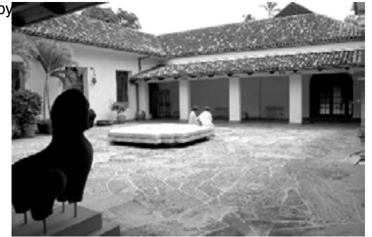
Image 11: The Banyan Court at the Honolulu Academy of Arts. Dacus, 2011. The double pitched roof sheltered windows and inhabitants from tropical sun and downpours. Library of Congress, Prints & Photographs Division. Photo by Chris Dacus, 2011.
