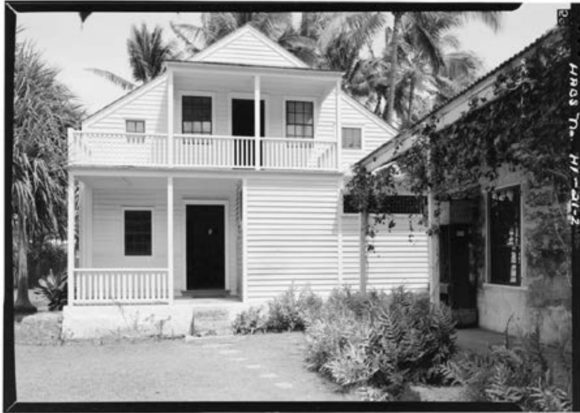
Image 2: West side of the Mission Frame House in Honolulu. The small windows and short eaves were inappropriate for the tropics as they provided little ventilation and protection from the sun and rain. However the later addition of larger windows and balconies helped adapt the buildings to Honolulu's climate. Photo courtesy of the Library of Congress, Prints & Photographs Division, HABS, Reproduction number. Photo by Jack E. Boucher.
