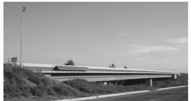
Fig. 1. Jamboree Road Over-crossing.
