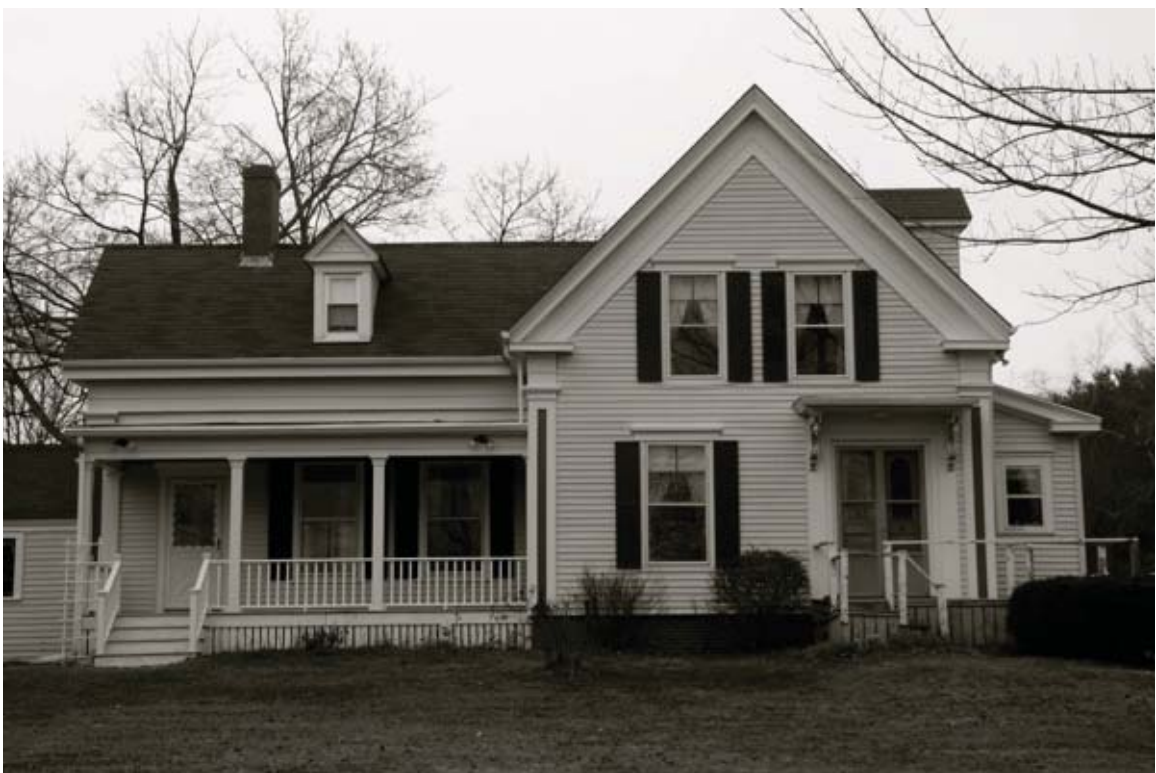
3-3. Chebeague home showing combination of Greek Revival and Italianate elements.
