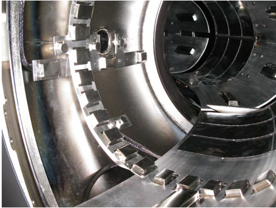
Figure 3.5: One section of the high-density toroidal array (upper left) after installation.
