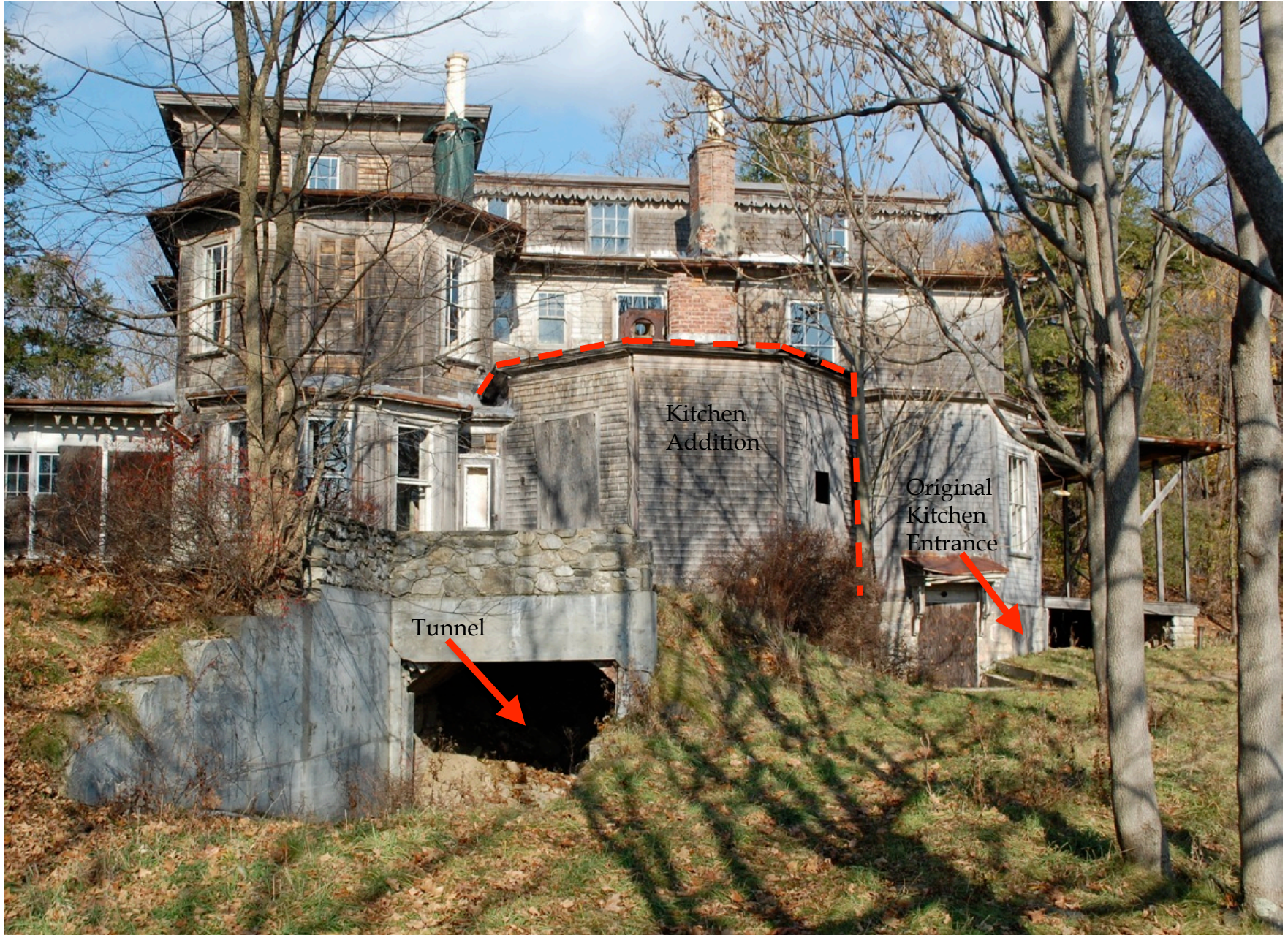
South Elevation of the Dr. Oliver Bronsohn House, November 2011. Image: Peter Watson.
