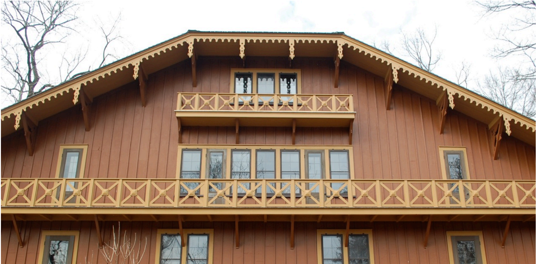
Detail of east elevation showing pair of doors in central window bank above balcony. Photo: Peter Watson.
