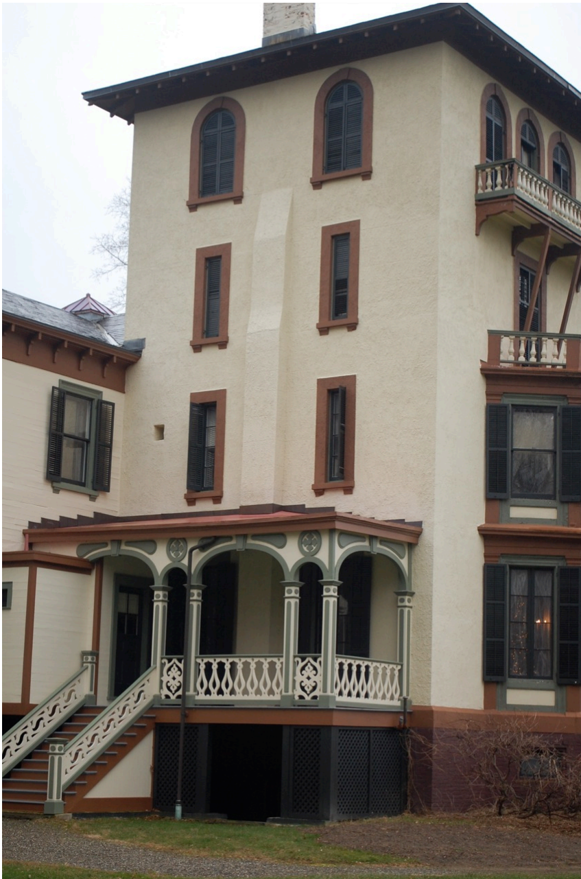
View of northwest veranda. December, 2011. Image: Peter Watson.
