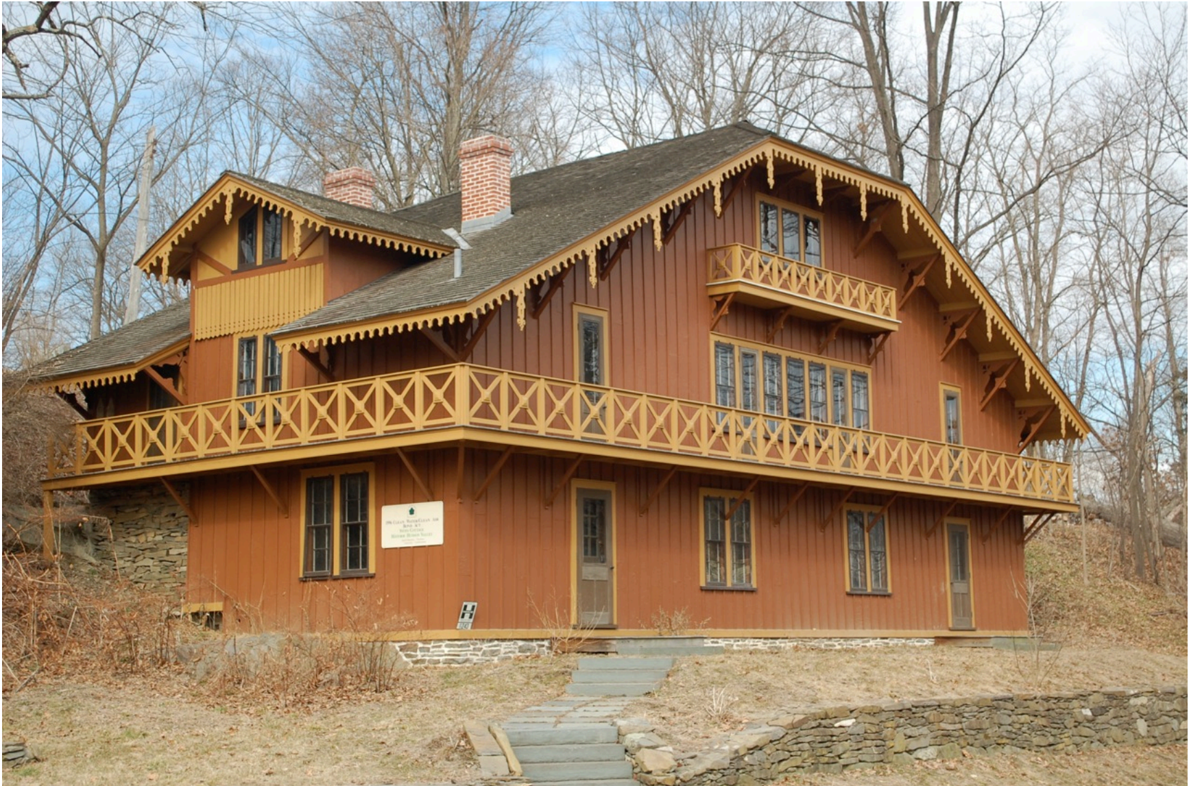
View of the Swiss Cottage from the southeast. Photo: Peter Watson.
