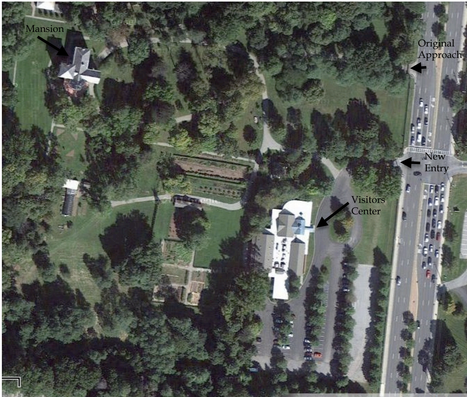
Aerial view of existing and proposed circulation at Locust Grove. Google Maps.
