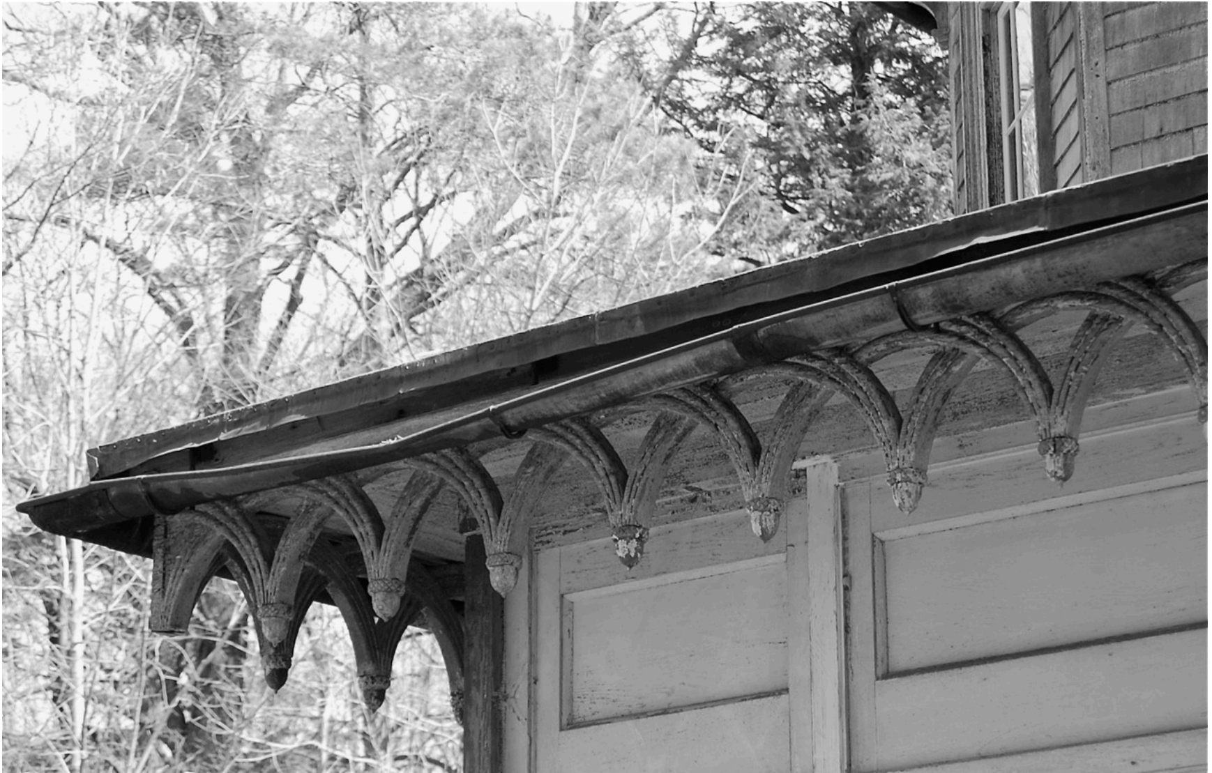
Dr. Oliver Bronson House. Detail of Norman arcading on west verandah. Peter Watson.
