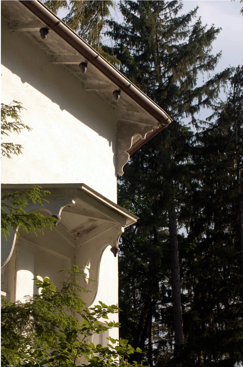
Detail of 1841 gate-house showing outlines of brackets. Image: Peter Watson.
