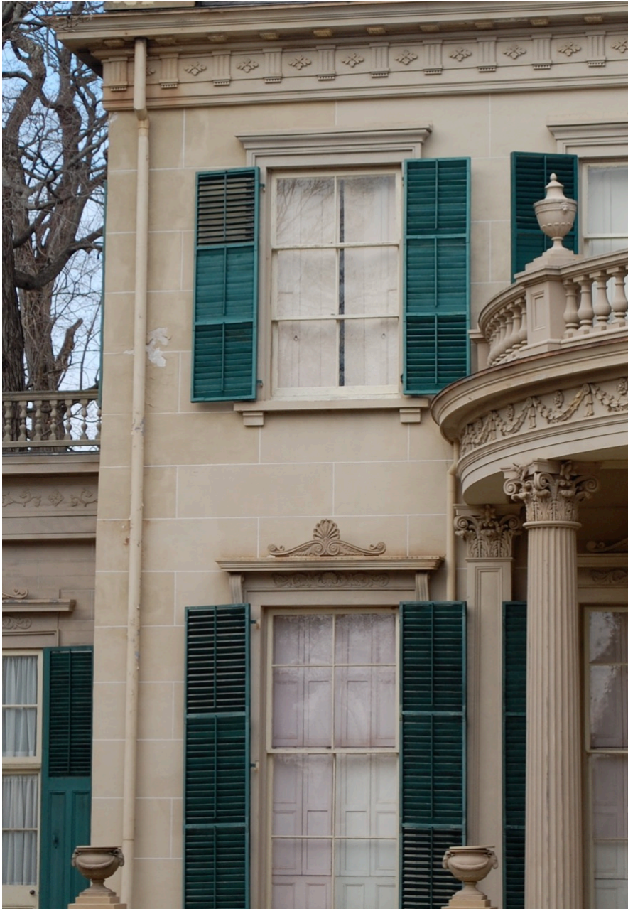
View showing differential treatment of first and second floor windows. Photo: Peter Watson.
