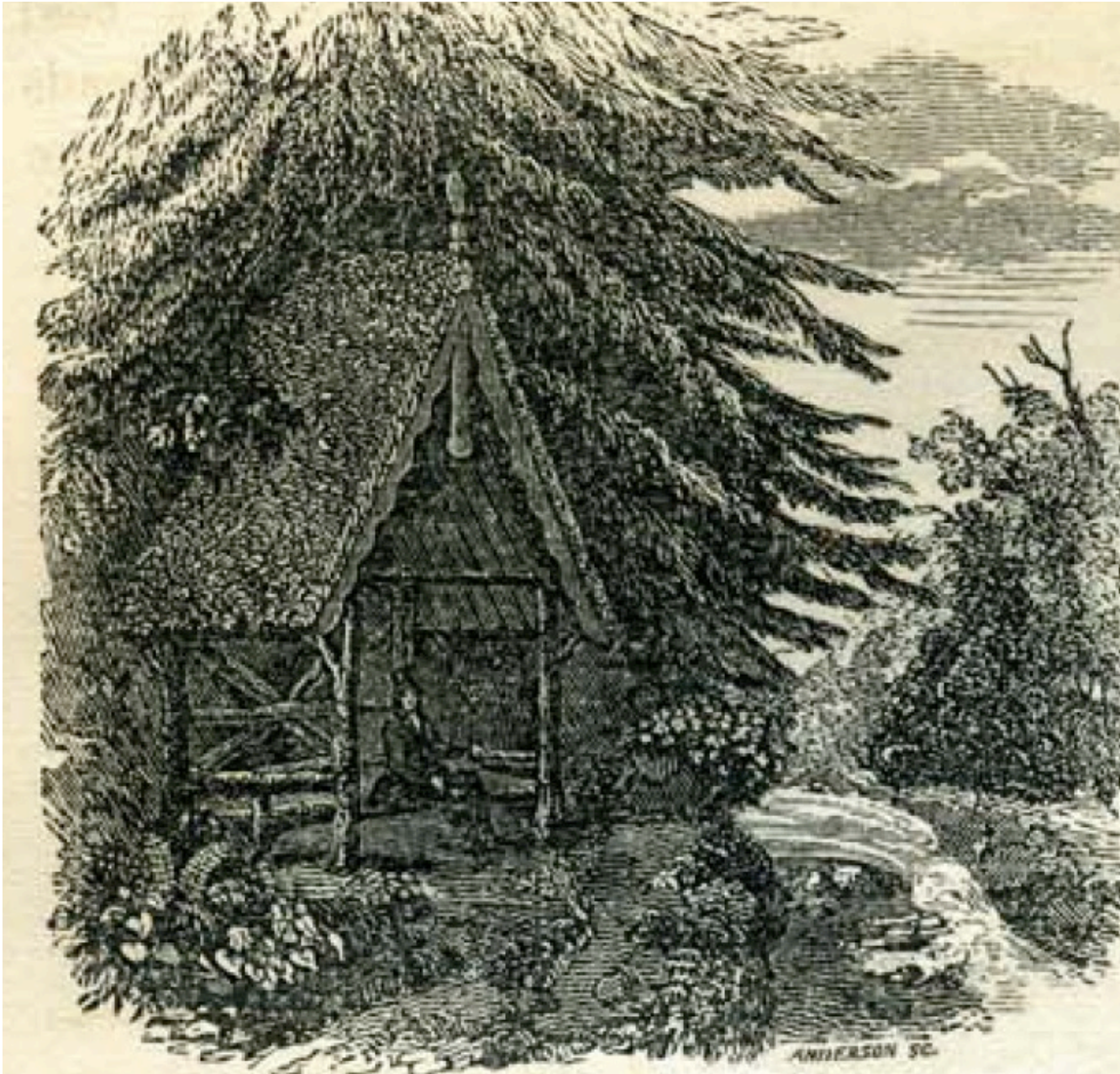
A.J. Davis. Rustic Shelter from "A Visit to Montgomery Place," The Horticulturalist , October, 1847.
