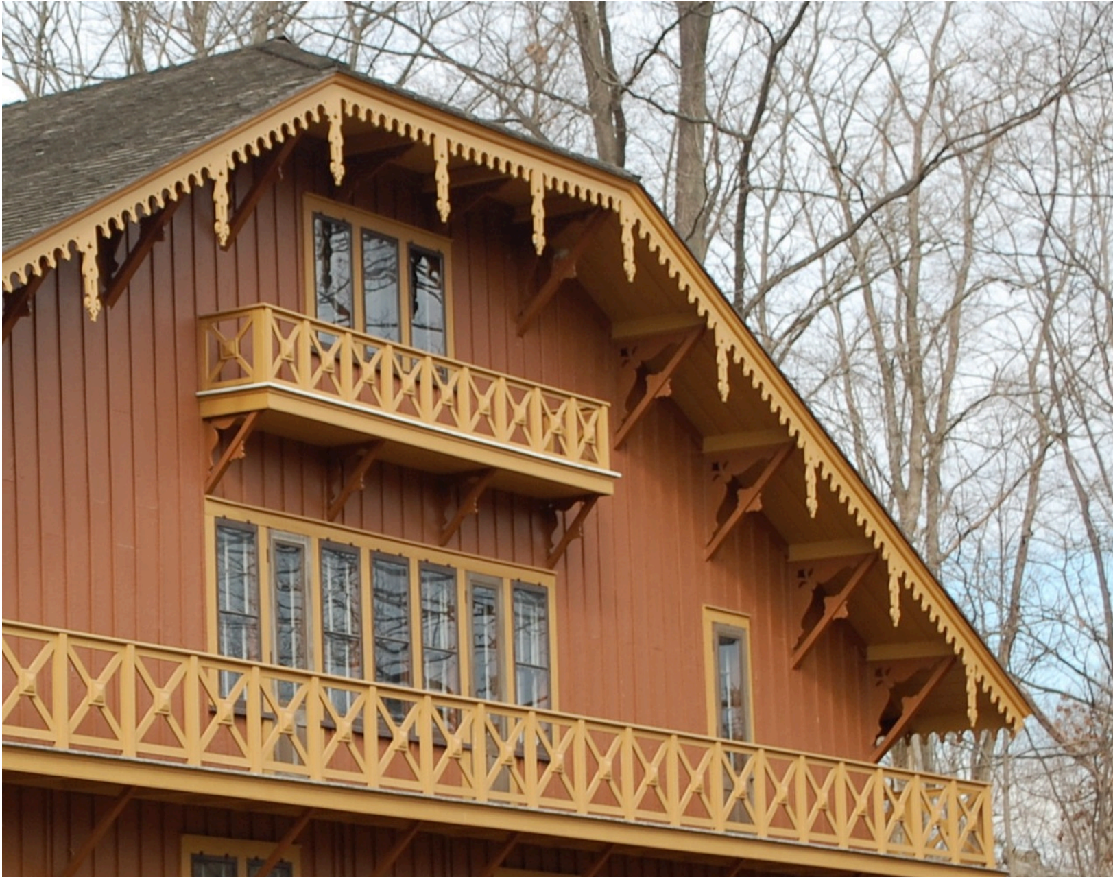
Detail of openwork brackets and ornamental drops on east elevation. Photo: Peter Watson.
