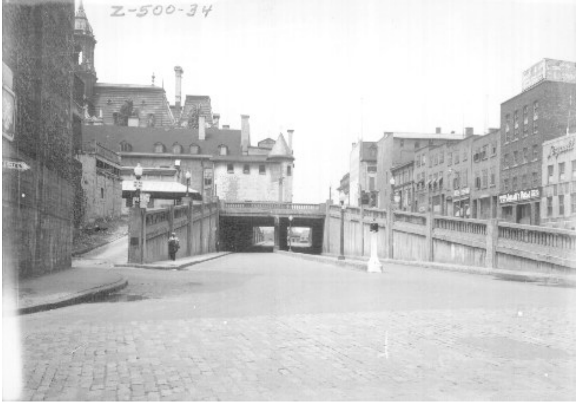
Figure 6. Gosford Tunnel underneath Chateay Ramezay, 1953 Archives de la Ville de Montréal VM94-Z-500-34
