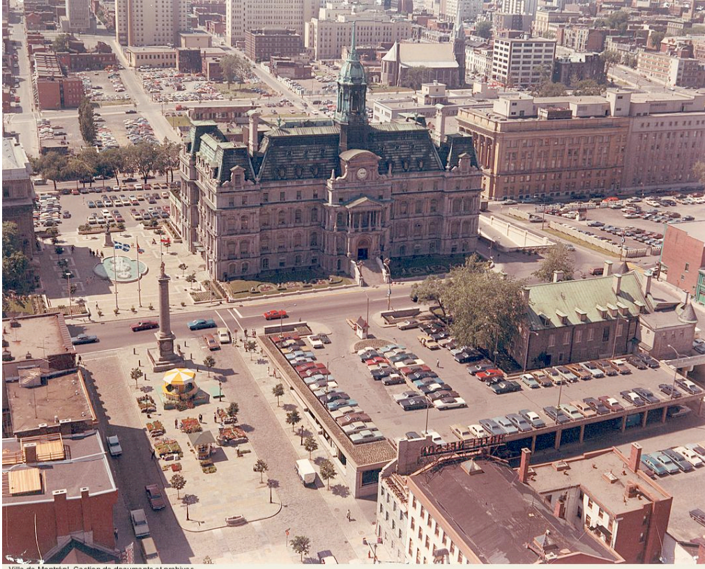
Figure 15. View north onto City Hall and environs, 1969 Archives de la Ville de Montréal VM6-S10-R3067-2-1-06
