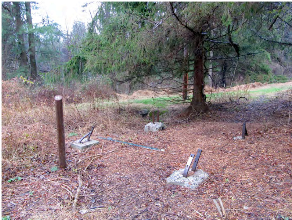
Figure 4-42: A stop at the foundation posts of a guard tower on the existing self-guided tour of Pine Grove Furnace, with subtle brown post marker on left (Rebecca Salgado)
