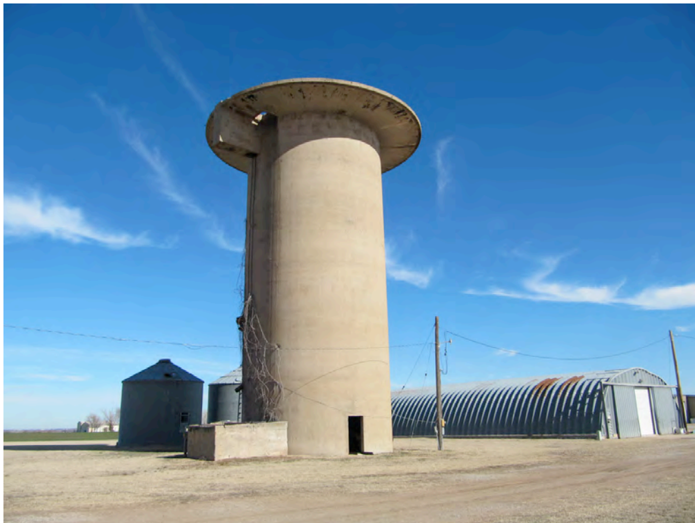
Figure 4-31: The remaining concrete water tower base from Camp Tonkawa; This tower can be seen in older views of the camp such as figures 22 and 23 (Rebecca Salgado)
