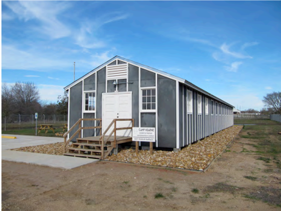
Figure 2-6: Camp Hearne's visitor center, constructed according to 1942 Army barrack plans (Rebecca Salgado)
