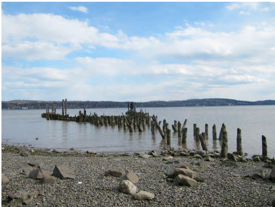
Figure 4-15: Dock remnants from the Camp Shanks era at the Piermont Pier (Rebecca Salgado)
