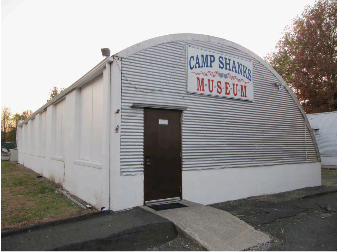
Figure 4-9: The exterior of the Camp Shanks Museum, located in a Quonset hut from the World War II era that used to be part of the Orangeburg Elementary School (Rebecca Salgado)
