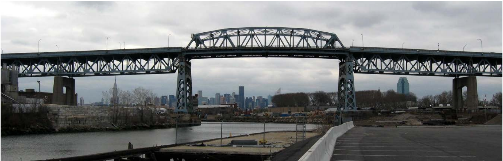
Figure 7-1 Kosciuszko Bridge over Newtown Creek
