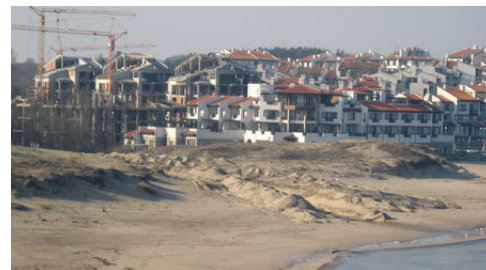
Construction on the old camp site Oasis
