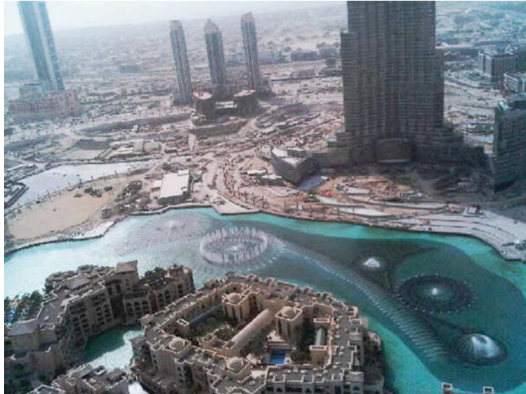
Figure 2. New development in Old Town Dubai, including the base of Burj Khalifa. Large development projects fail to produce an articulated urban fabric and demonstrate unsustainable use of water in the desert city. Photograph: Ameera Akkila.
