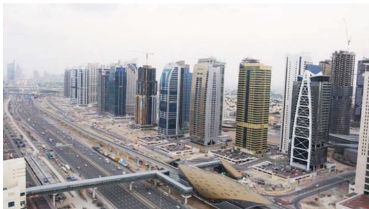
Figure 5. Metro line along Sheikh Zayed Road. Photograph: Alamira Reem Bani Hashim.
