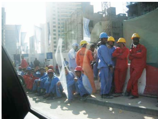
Figure 8. Labourers on construction site. Photograph: Ahmad Huzair.
