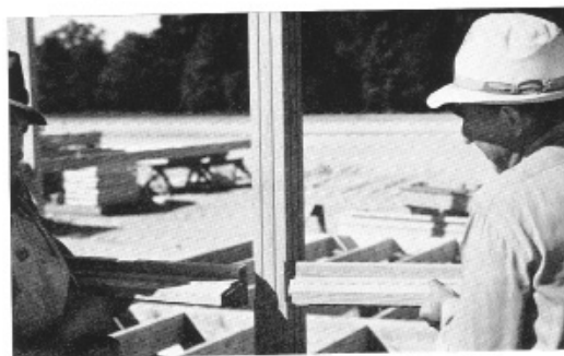
The window course sills fit into recesses in the wood columns. The sills are also a millwork product.
