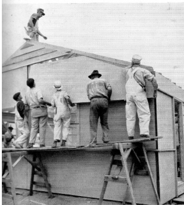
A Cemesto Board gable is installed.
