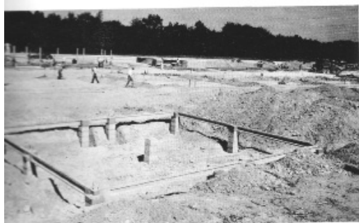
Each house rests upon concrete piers and precast concrete rails.
