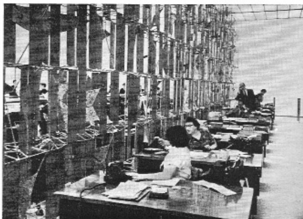
MASSIVE SCREEN on second floor was designed to break up floor expanse without interfering with the circulation of air. Critics likened it to an old scaffolding.
