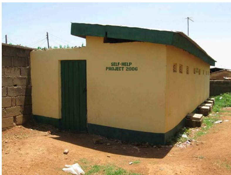
Figure 7: Photo of Toilet Block Constructed in 2006
