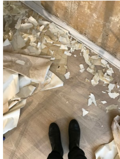
Picture 92: Renovation in the store, Daria Ivanova 2017
