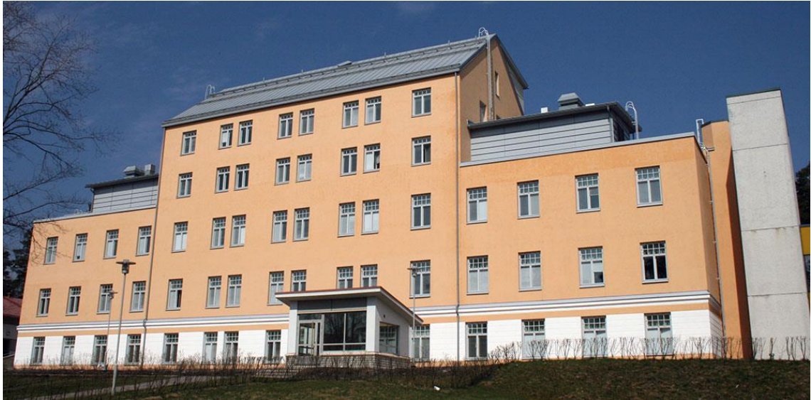
Figure 5. Keratam Oy's plastering project picture
