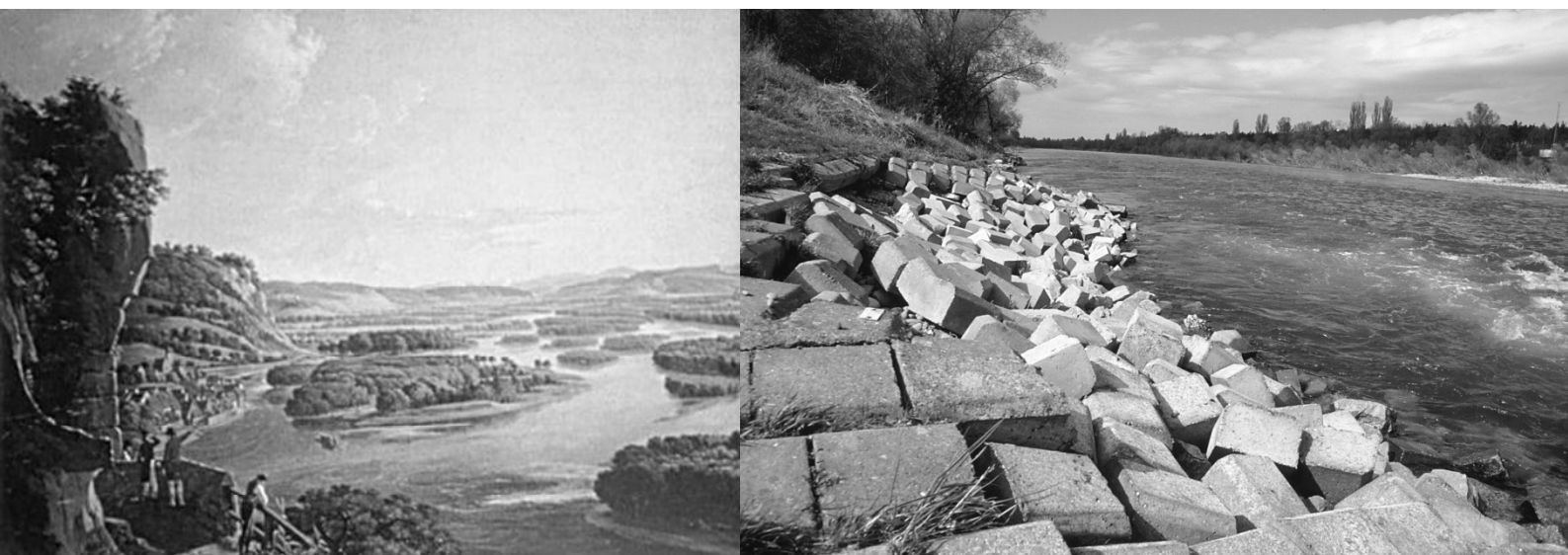
Figure 1.3 The Rhine River between Basel (S) and Karlsruhe (D) was regulated in the 19th century by the German engineer J.G. Tulla. An island dominated river of 5 km wide (left) was canalised, leaving a single small navigable channel in the present Restrhein (right; photo G.W. Geerling).
