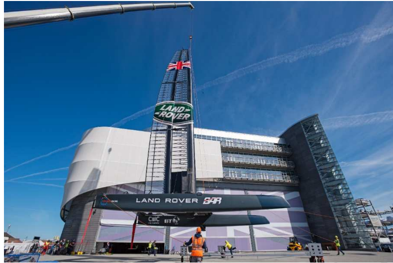
Figure 2a. External view of the new Land Rover Bar Team HQ building from the west. Showing yacht being craned out to the sea. The sea is on the immediate left of the photograph
