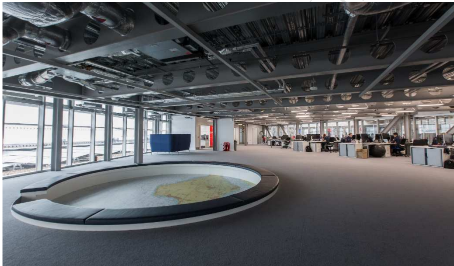
Figure 2d. View of the office floor taken from the south east corner
