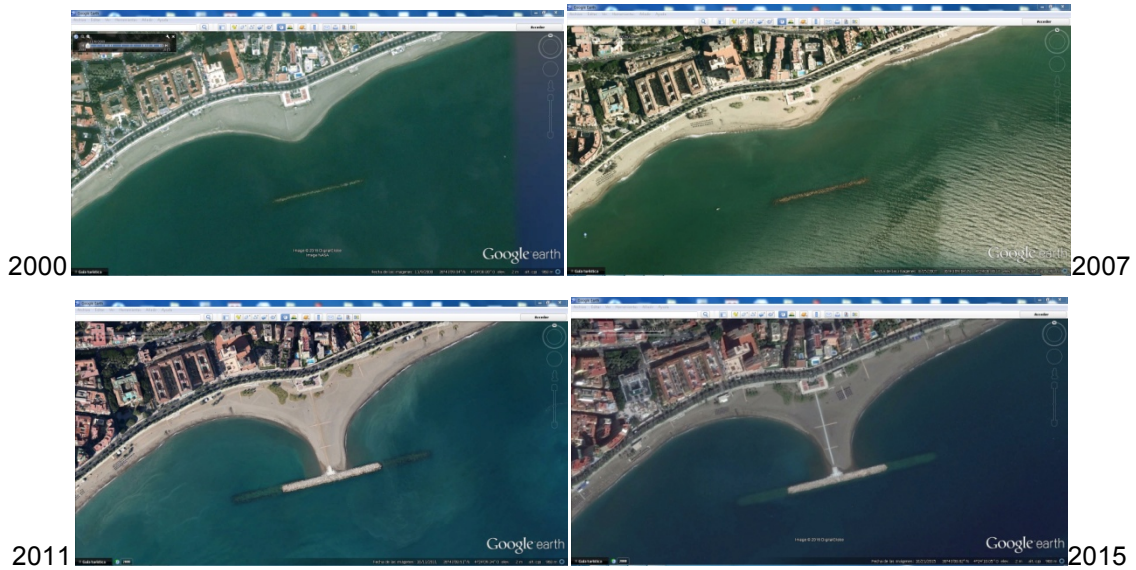
Fig. 6. Example of Breakwater in Malagueta Beach (Málaga, Spain).
