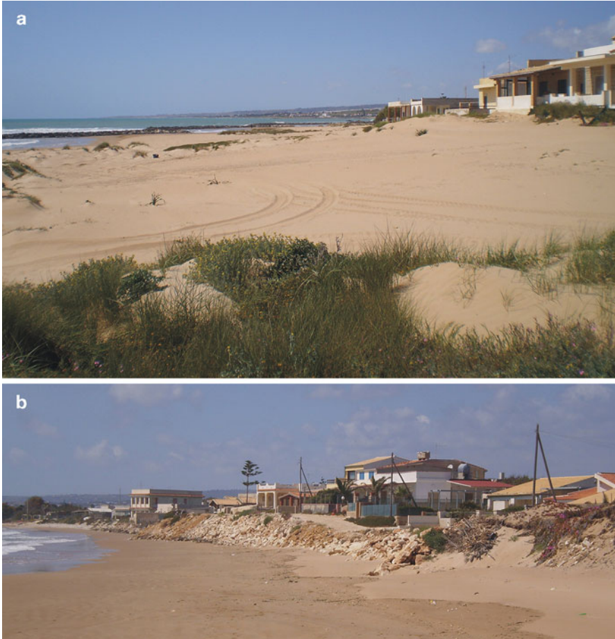
Fig. 13.6 Migrating dunes at the northern breakwaters emplaced downdrift (east) of Donnalucata harbour (a, April 2011); summer houses protected by rip-rap revetments downdrift (east) of easternmost breakwater at Modica Stream mouth (b, April 2011)
