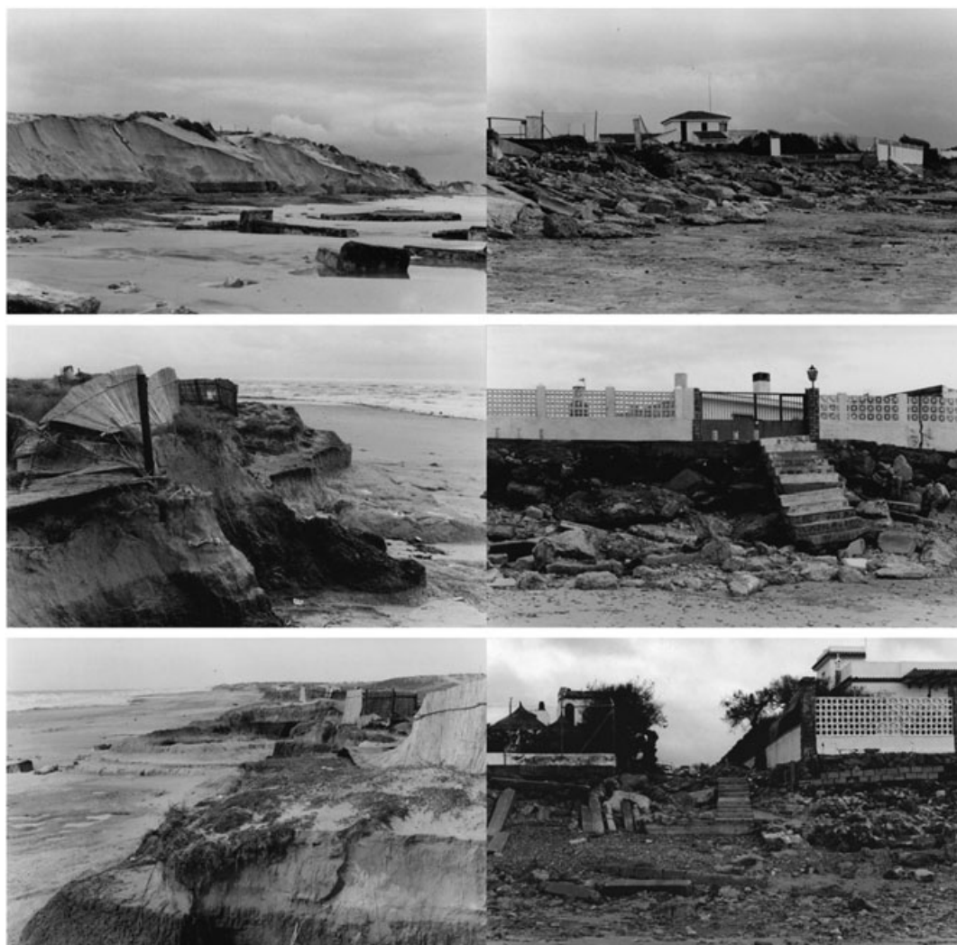
Figure 8. Examples of dune and cliff erosion (left side) and beach damages (right side) along the Peginas and Punta Candor areas associated with the impacts of storms over the 1995–1996 winter period (storm events T6–T12 in Figure 9).
