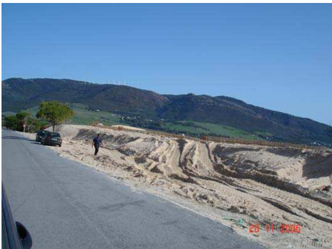
Figure 3.- A Punta Paloma road view after dune works
