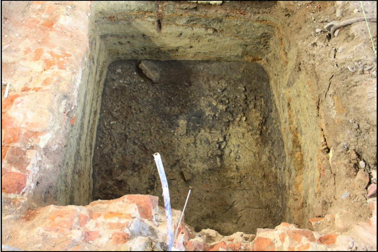
Figuur 74: Keienniveau in liftput 2.
