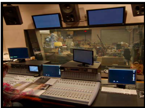
Figura 10. Control Room. Extraído de Wbsound.com
