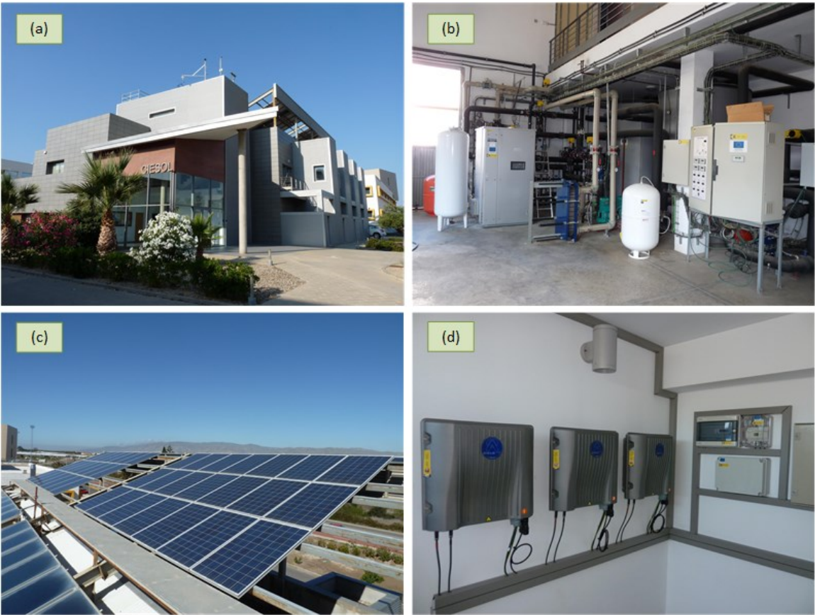
Fig. 6.1. The CIESOL building: (a) Exterior of the CIESOL building; (b) Solar cooling installation; (c) Photovoltaic power plant: PV panels; (d) Photovoltaic power plant: PV inverters.
