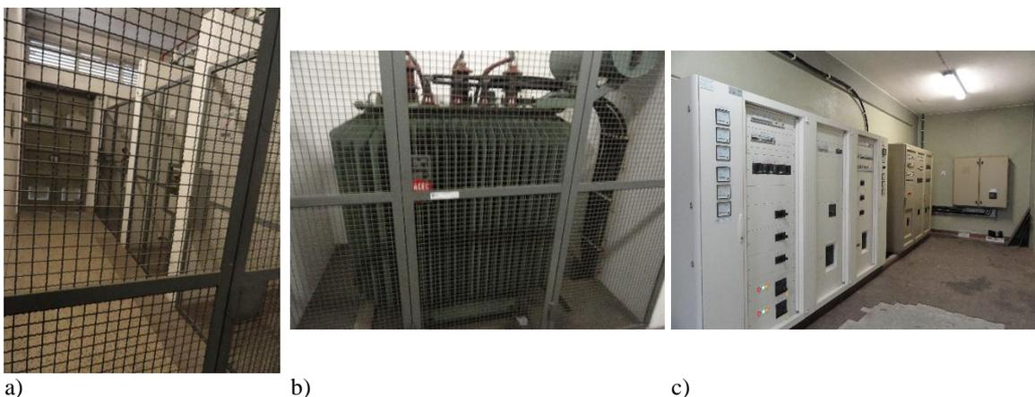
Figura 4.7 – a) Celas EDP; b) TP<sub>2</sub> do PT<sub>1</sub>; c) QGBT e BC do PT<sub>1</sub>
