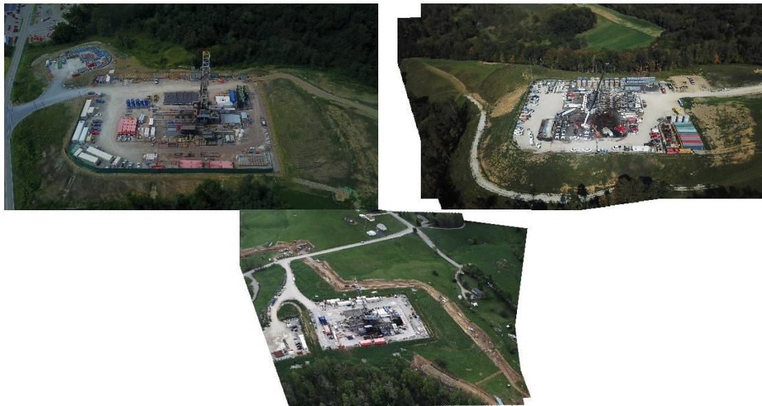
Figure 3. Examples of a typical hydraulic fracturing well pad in Eastern Ohio including a record breaking lateral pad at the Walleye Pad (Top-Left).
