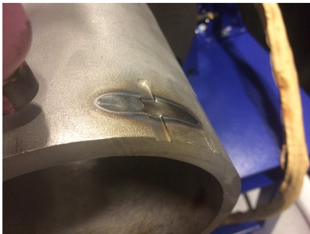
Fig. 7: Picture of one of the introduced notches Post-Welding.
